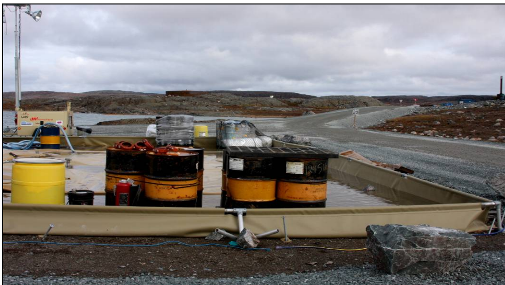
Figure 5. Fuel transfer station with fuel transport pump contained within a berm at Robert Bay
