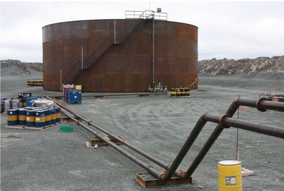
Figure 3. Fuel Tank (5 million liter) at the former Quarry #1 site near Roberts Bay
