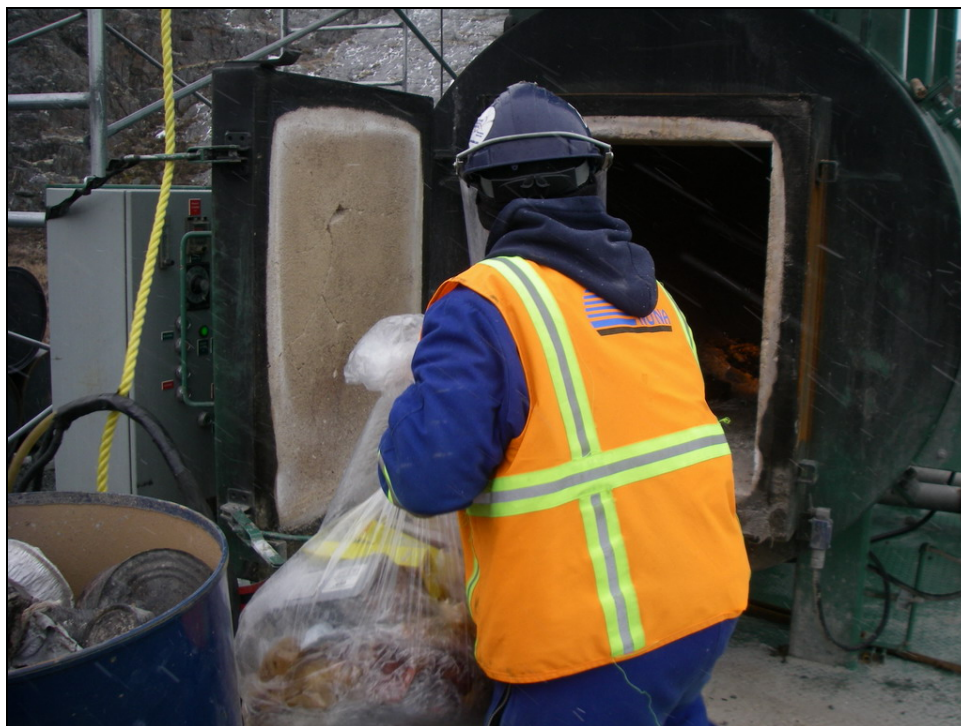
Plate 2.1-3. The incinerator operator adding waste to the Doris incinerator primary chamber, September 2009.
