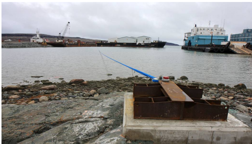
Figure 4. Land based mooring point
