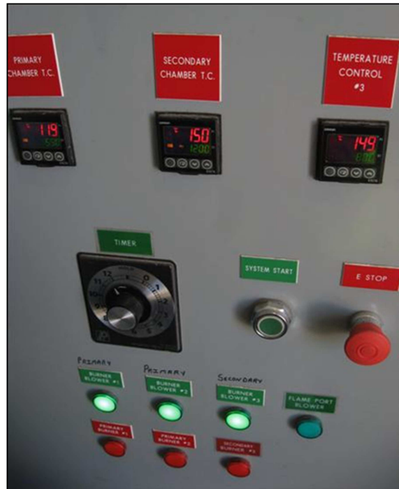
Plate 2-4. There are three digital temperature readings displayed on the upper row. The lower light display shows the function of the secondary and primary burners and blowers.
