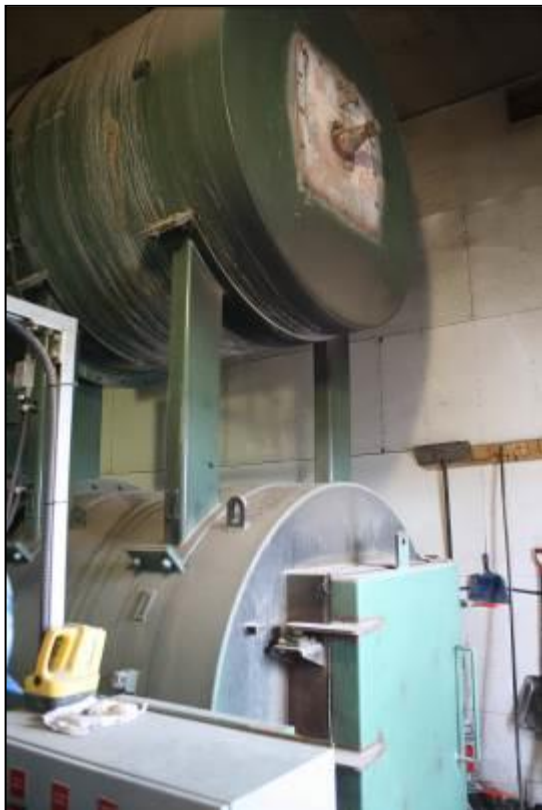
Photo 7: Incinerator
