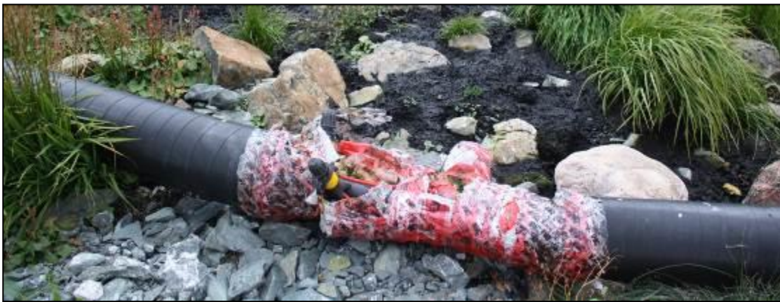
Photo 10: Wildlife tampering along sewage pipeline
