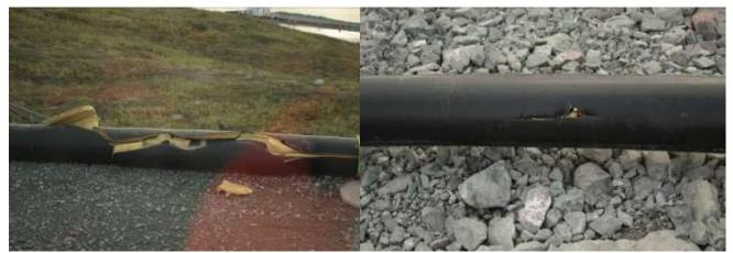
Photo 42 – Cracked insulation on TIA line adjacent to water intake
