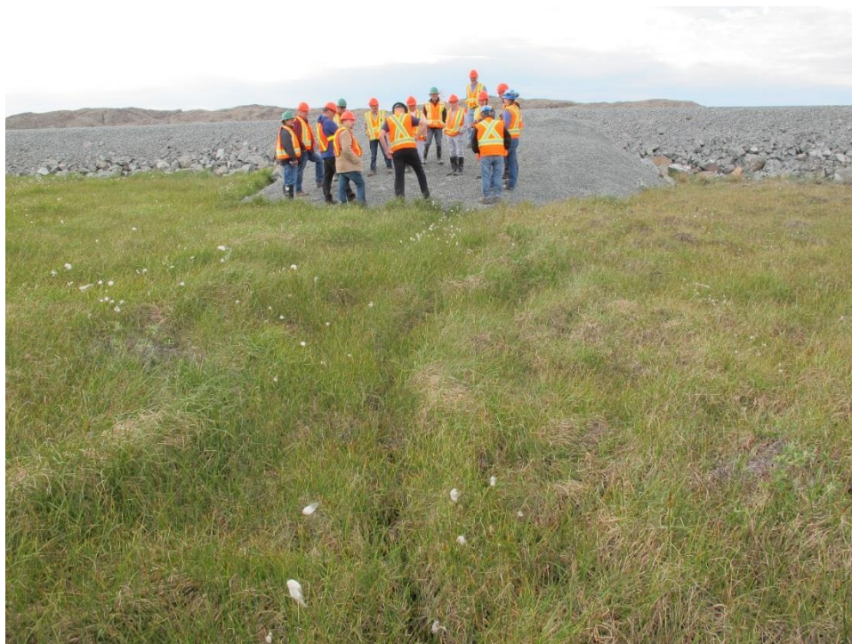
Plate GN-19-1. Caribou trail leading to road crossing structure for the existing Doris to Madrid road.
