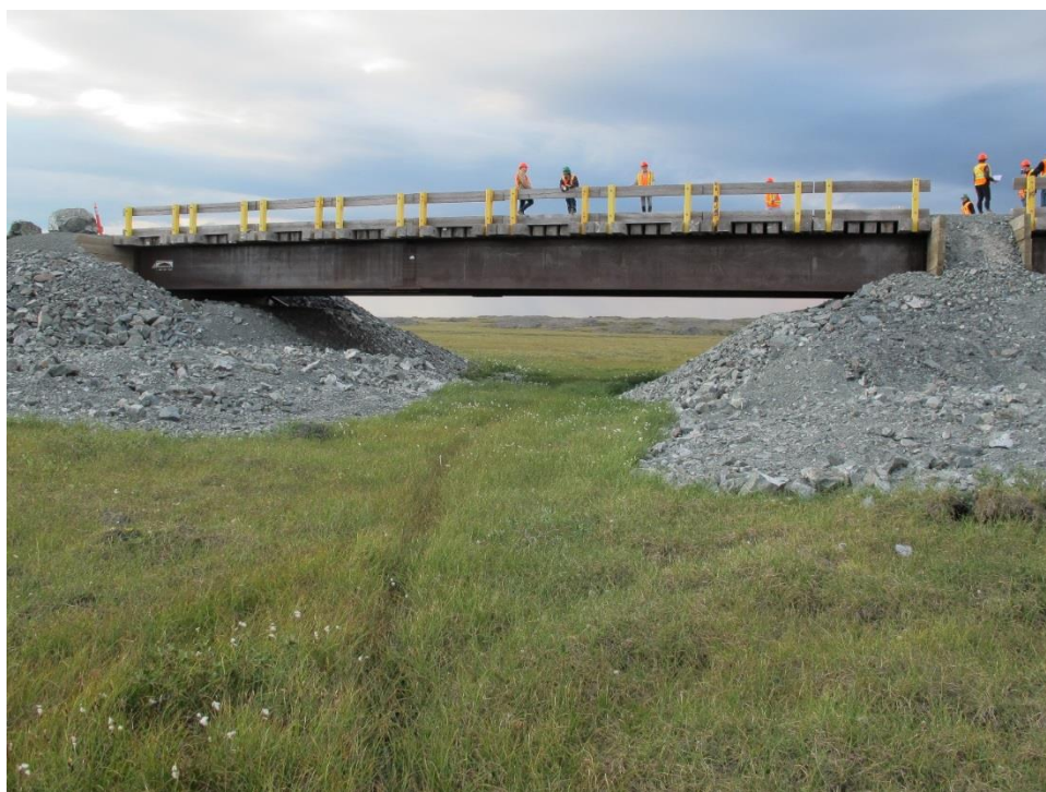
Plate GN-10-2. Caribou trail leading under the bridge over a wetland area on the Doris to Madrid road.
