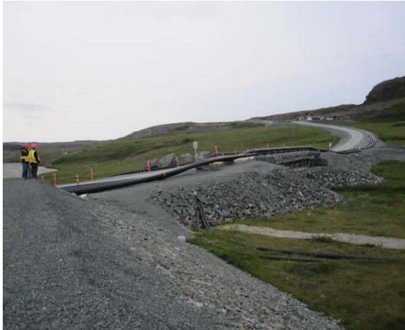
Photo 25 - Tailings and reclaim water pipelines
