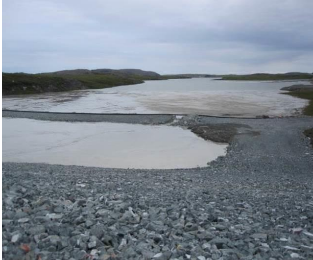
Photo 34 - Newly constructed cofferdam in the south end of the Tailings Impoundment Area
