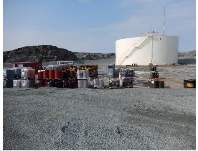
Photo 42 - Fuel storage tank and fuel drums in a lined and bermed secondary containment area at Roberts Bay
