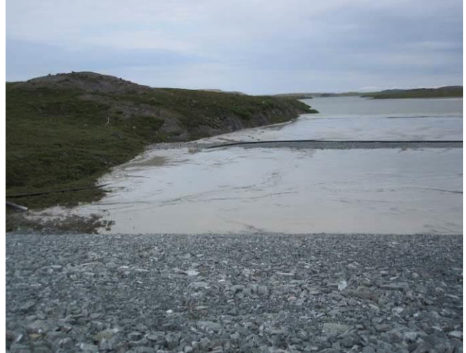
Photo 35 - Outfall/spigot for tailings discharge in the south end of the Tailings Impoundment Area
