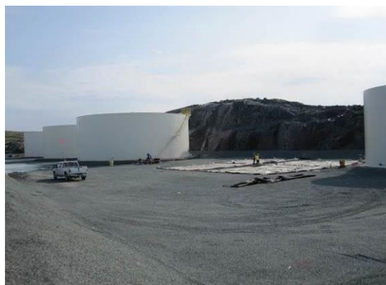
Photo 3 -Fuel Bladder Storage System at Roberts Bay Tank Farm
