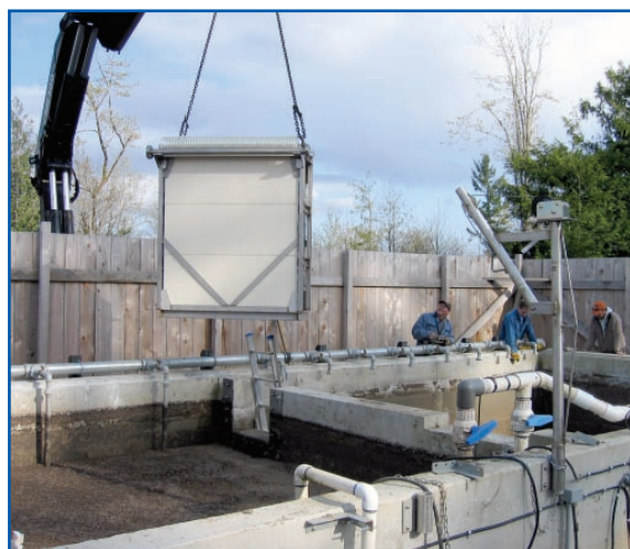
SaniBrane® flat-plate unit being installed in a concrete tank.
