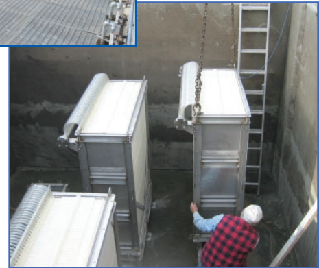
Installing the MBR units.
