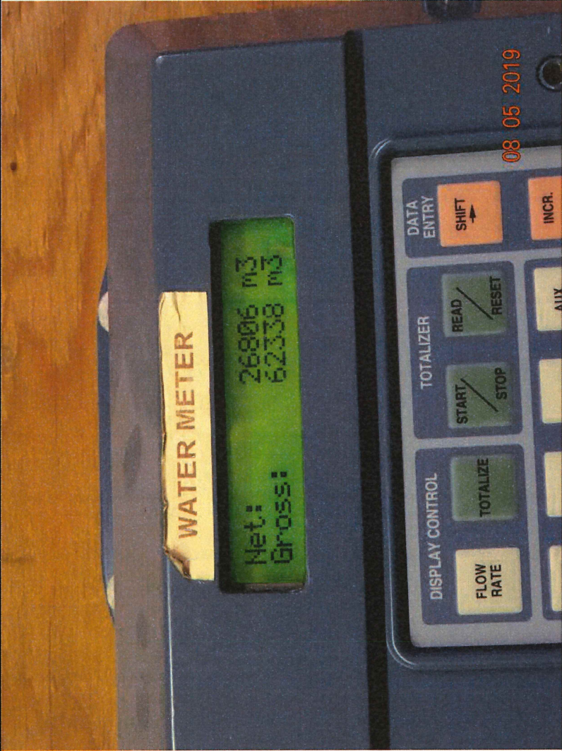
Description: Flow meter at the Raw Water Intake Facility
