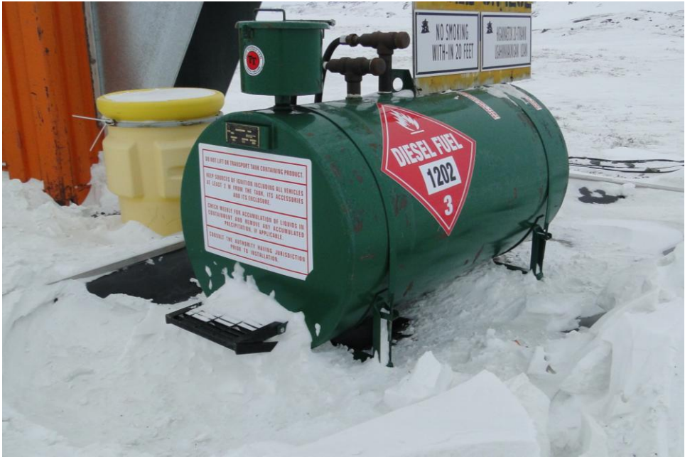
Tank for backup generator at Water Pump House – berm full of snow.
