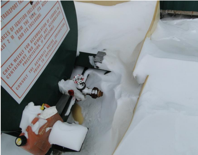
Berm under tank at heli-pad. Wall is torn and berm is full of snow.
