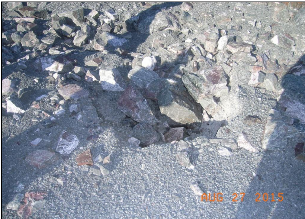
Photo: 3.8-4 Quarry #1 Overburden Dump; area of subsidence
