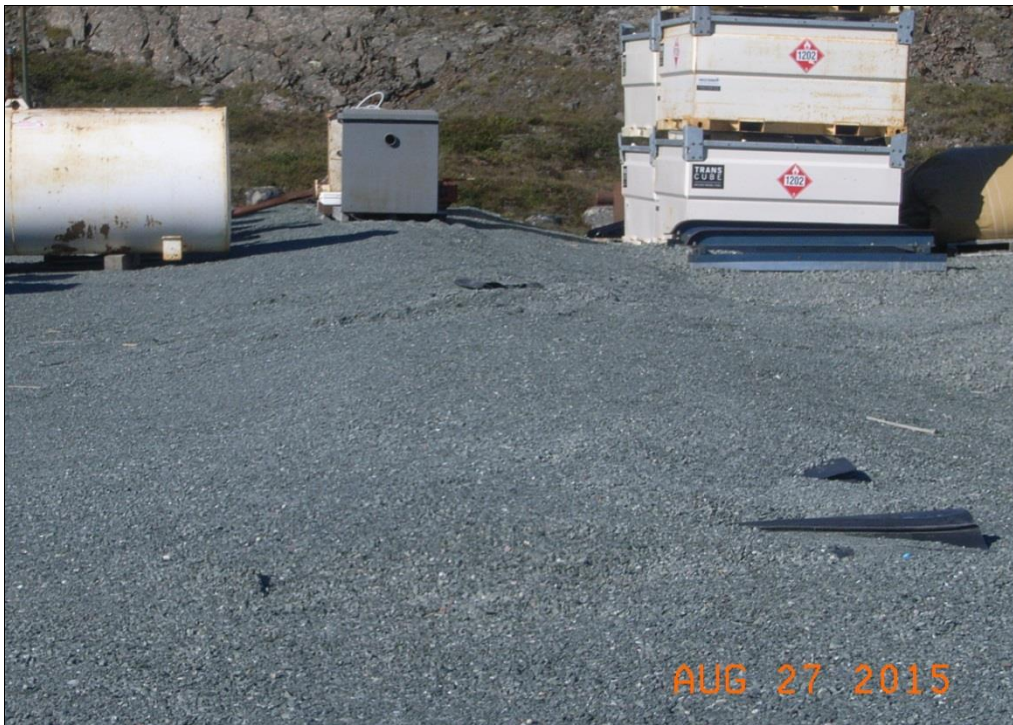
Photo: 3.12-2 Upper reagent pad AN secondary containment bund; exposed HDPE liner
