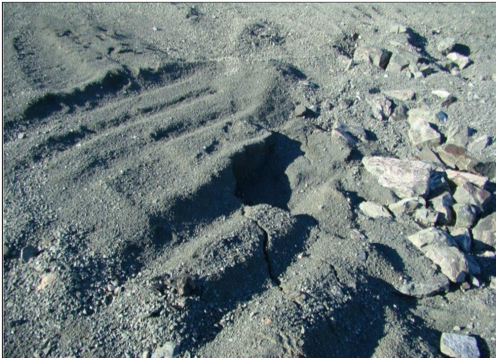
Photo: 3.8-1 Quarry #1 Overburden Dump; area of subsidence
