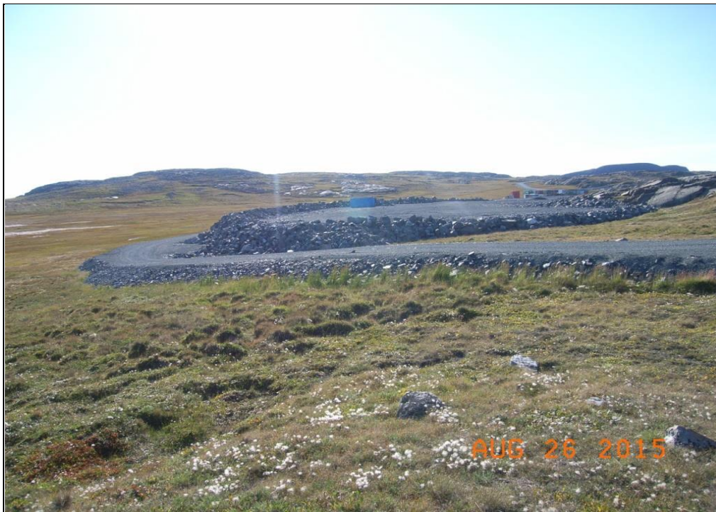
Photo: 3.8-2 Quarry #1 Overburden Dump; surrounding sediment control berm
