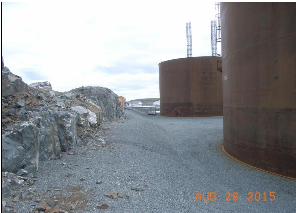
Photo: 3.19-4 Doris North Tank Farm; containment bund and rock cut
