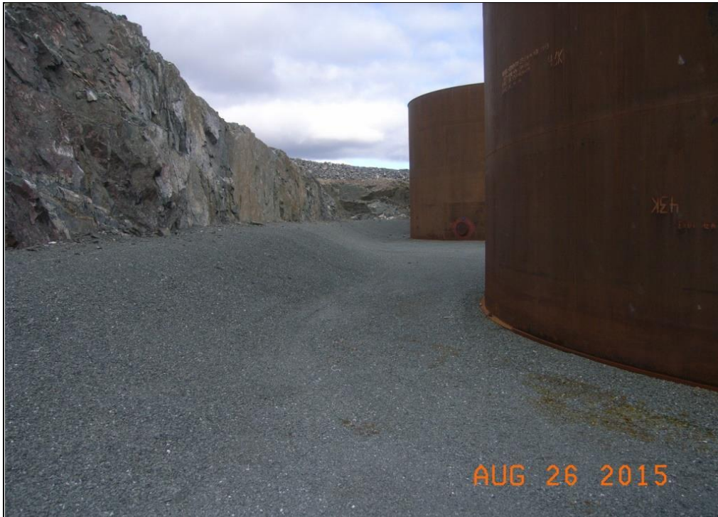
Photo: 3.19-3 Doris North Tank Farm; containment bund and rock cut
