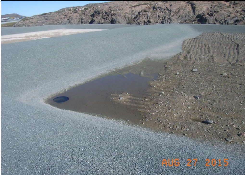
Photo: 3.15-3 Landfarm; sump in soil cell
