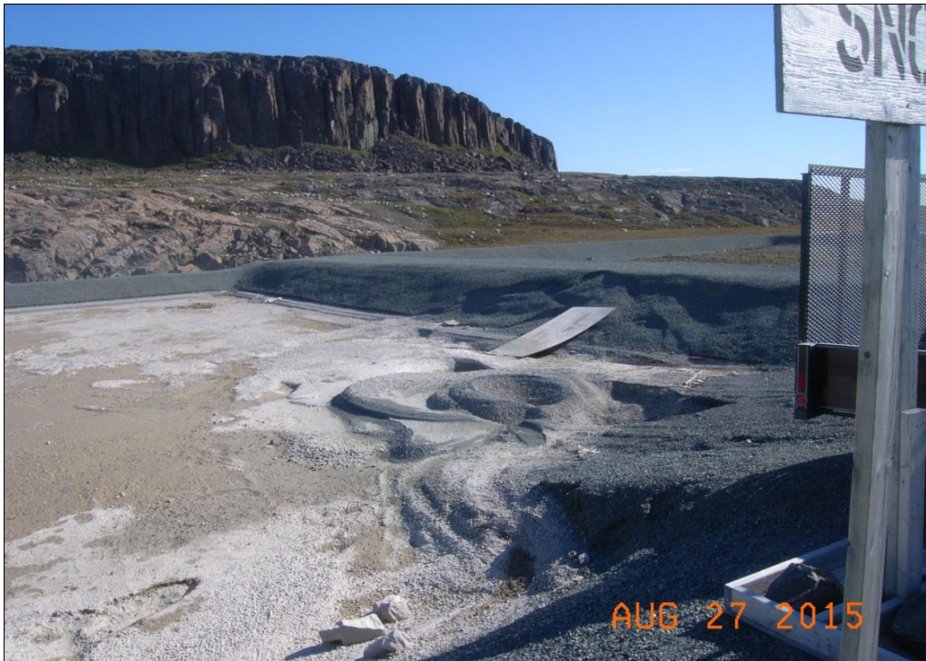
Photo: 3.15-5 Landfarm; snow cell – damage to internal ramp
