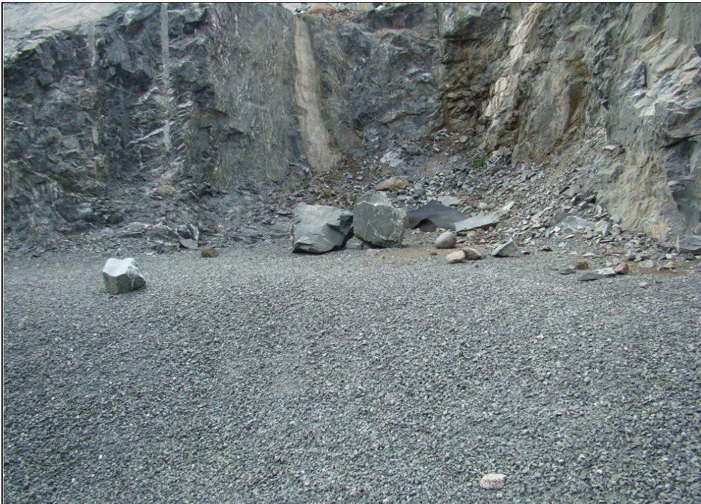
Photo: 3.19-2 Doris North Tank Farm; containment bund; fallen rock pieces on top of containment bund
