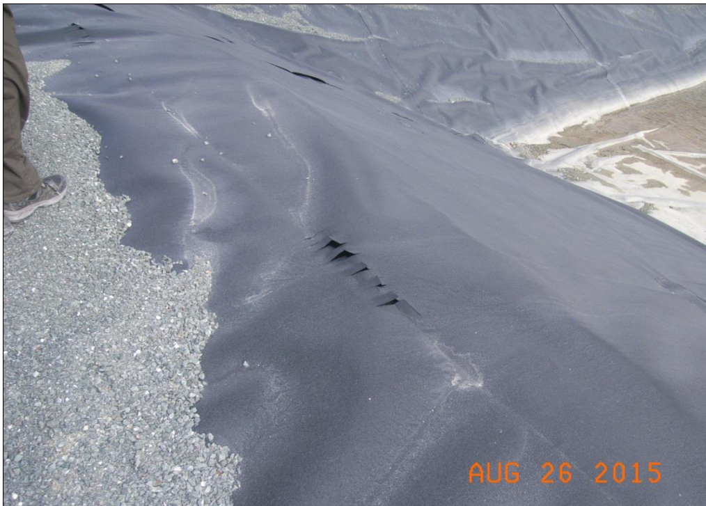
Photo: 3.24-4 Sedimentation Pond; cuts in HDPE liner
