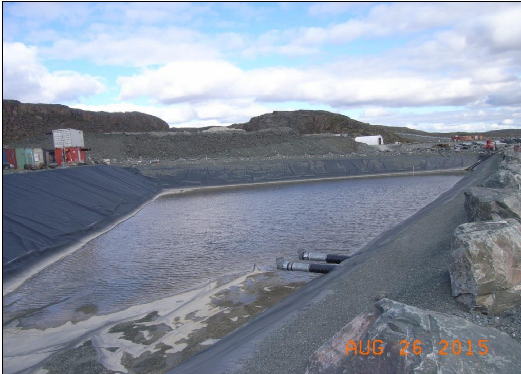
Photo: 3.24-3 Sedimentation Pond; HDPE liner and overflow pipes
