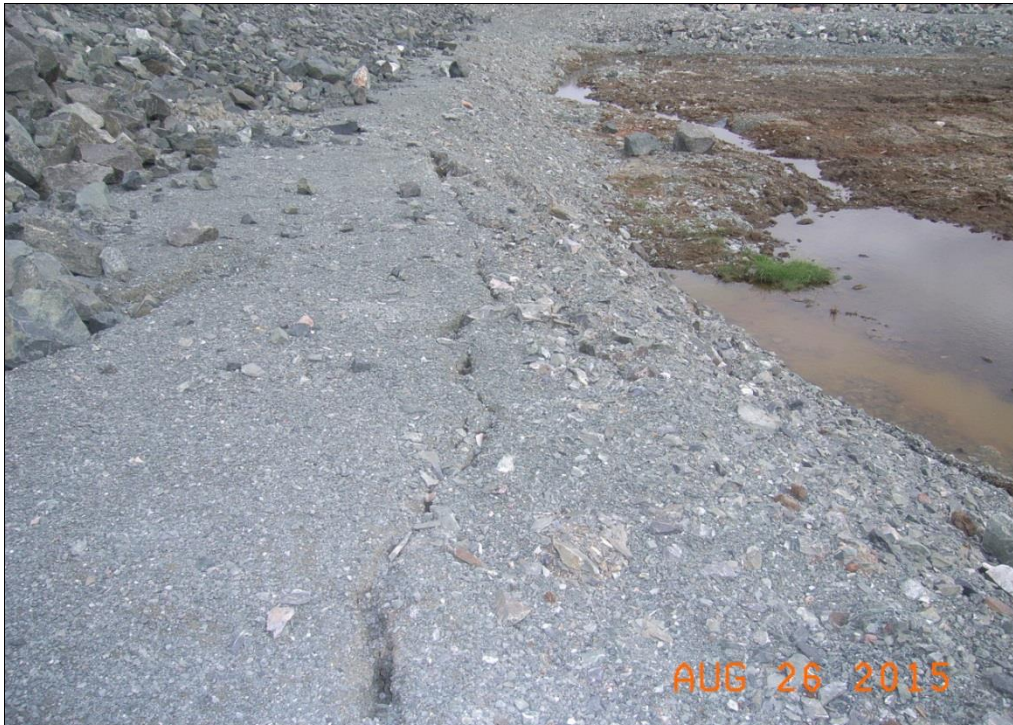
Photo: 3.24-2 Pollution Control Pond – tension cracks
