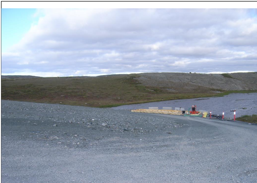
Photo: 3.30-5 Doris North Dam; depression along up stream slope face and pumping equipment at toe
