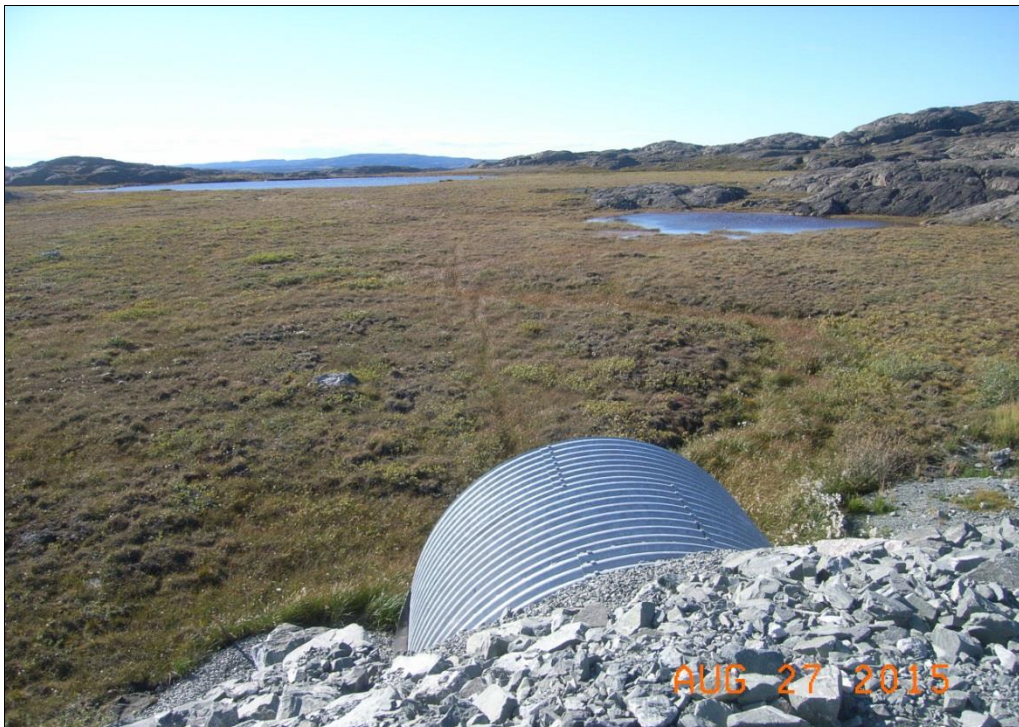
Photo: 3.34-2 Doris-Windy All- Weather Road; Stream Crossing #1 arch culvert
