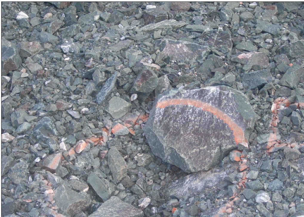
Photo: 3.30-6 Doris North Dam; depression along downstream slope face
