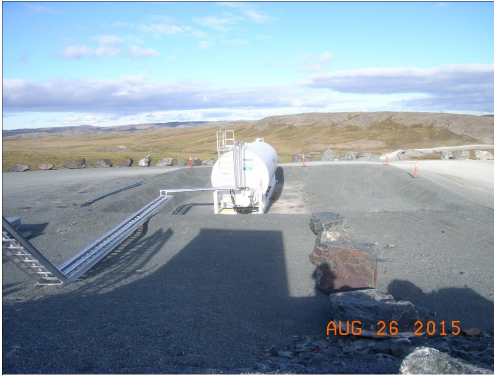
Photo: 3.28-3 Doris Primary Vent Raise Pad; fuel containment bund
