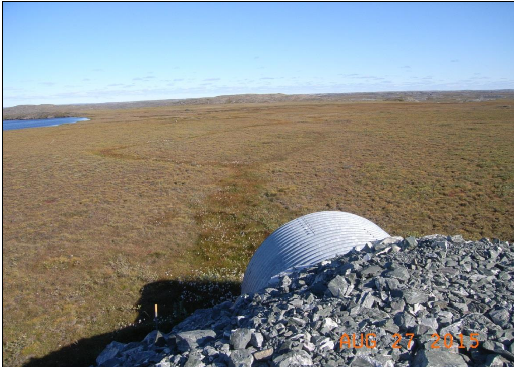
Photo: 3.34-1 Doris-Windy All- Weather Road; Stream Crossing #1 arch culvert
