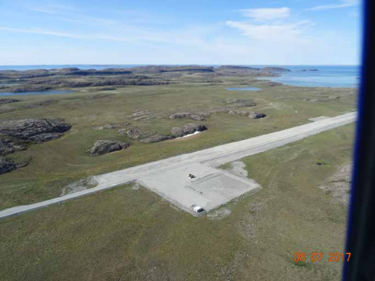
Description: Aircraft de-icing pad (under construction). Liner will be present to contain the fluid. No sediment control measures noted.
