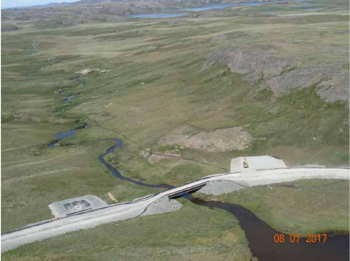
Description: Catchment basins on either side of Doris Creek. East basin was under construction at the time of the inspection.
