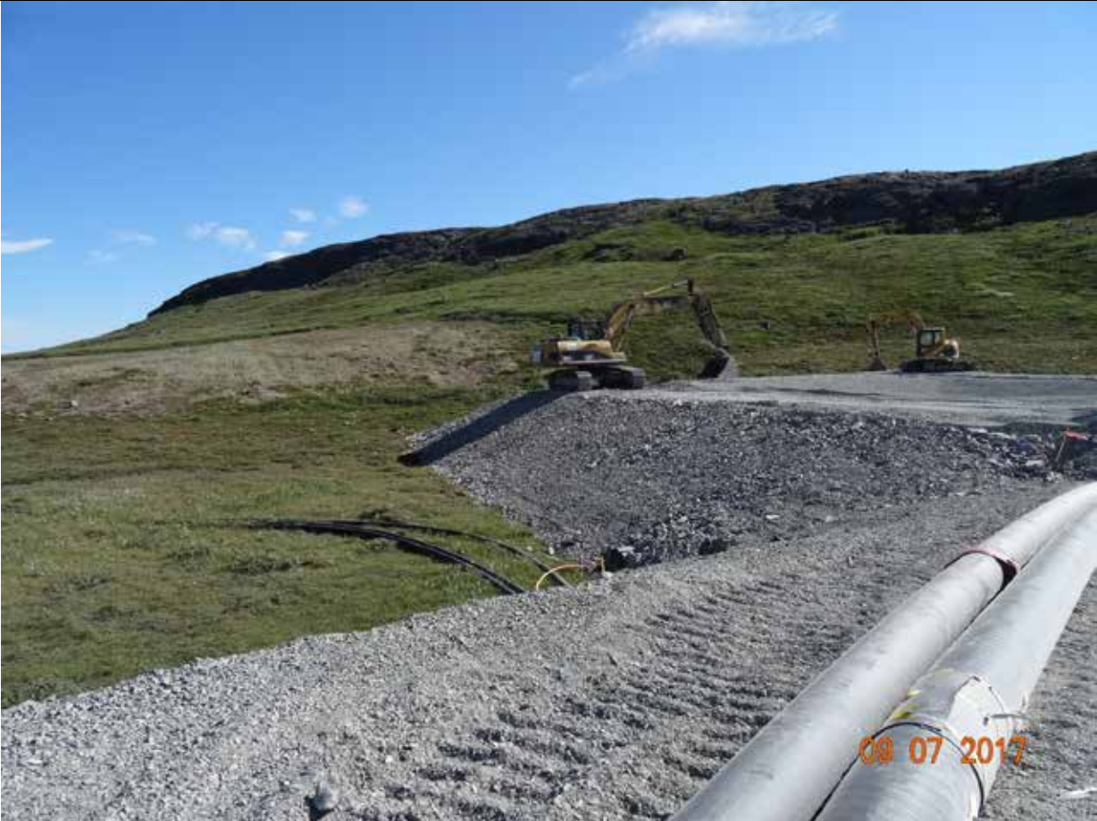
Description: East catchment basin; no sediment control measures in place.
