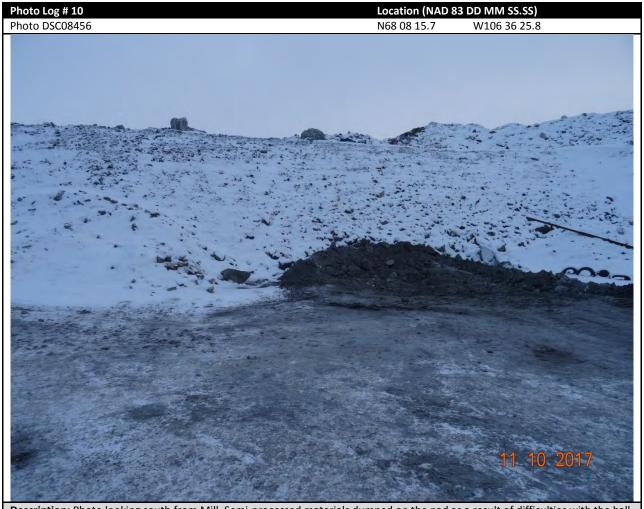
**Description:** Photo looking south from Mill. Semi-processed materials dumped on the pad as a result of difficulties with the ball mill.
