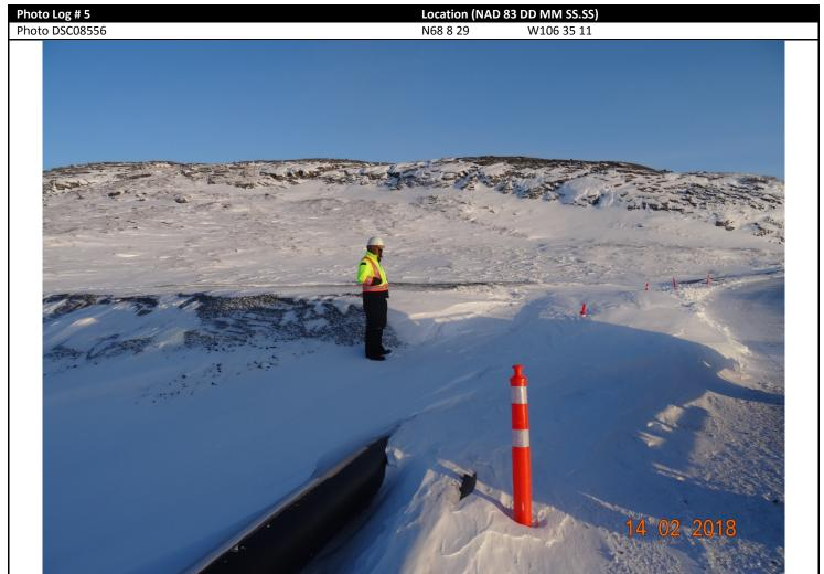
Description: Emergency Catch Basin on west side of Doris Creek. The Tailings pipe is under snow along the orange pylons with no indication of direction into Basin if necessary.
