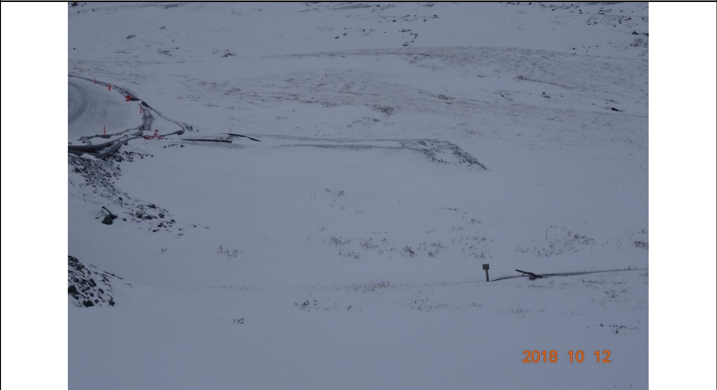
Description: east catchment basin closer to the vent raise. Slumping can be seen through the snow cover.
