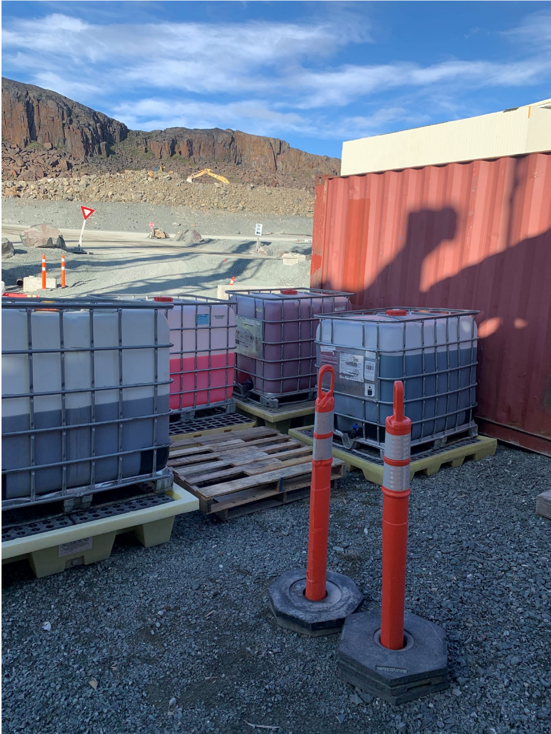
Photo 2 : Totes at the powerhouse placed on a secondary containment
