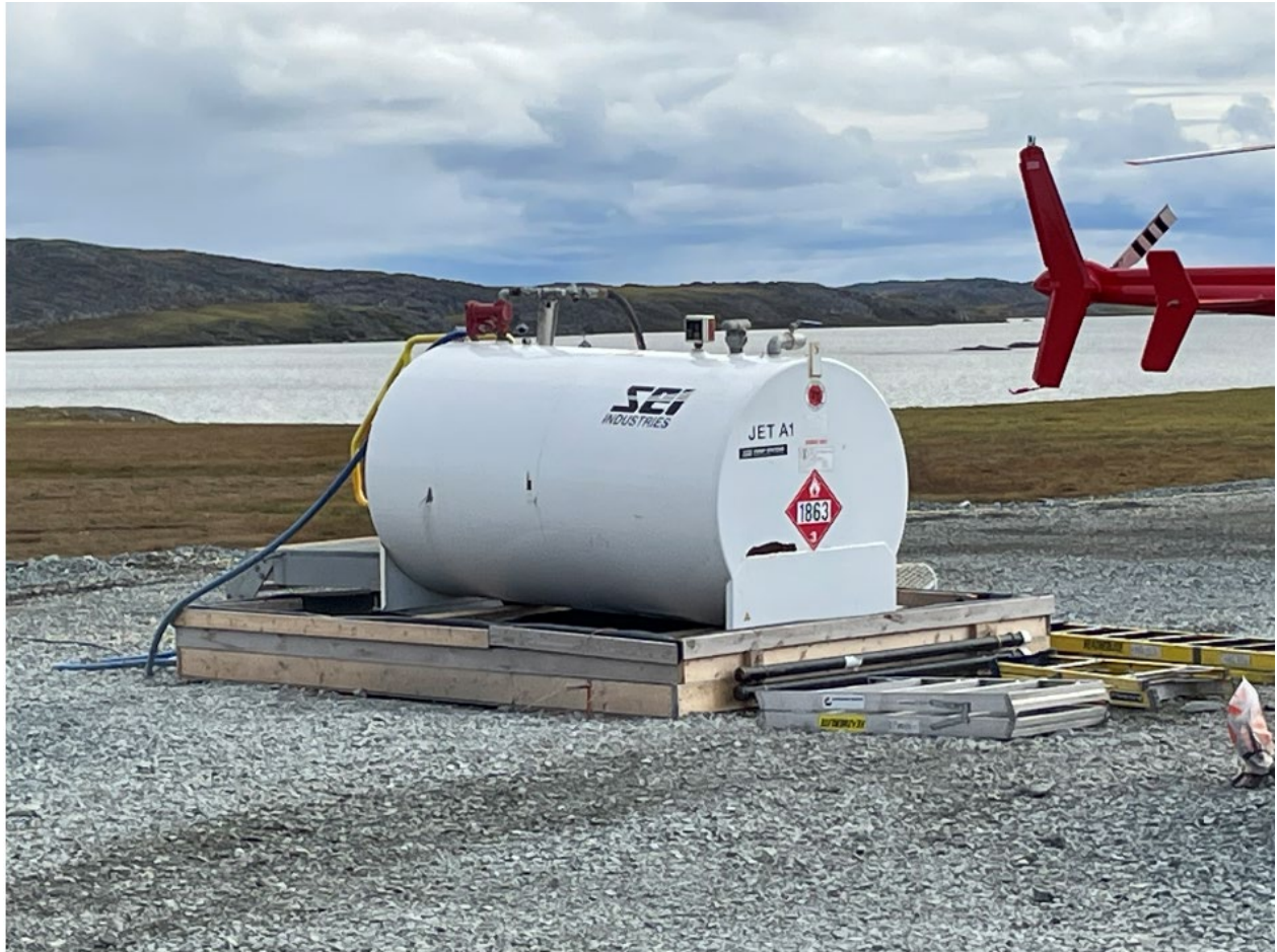
Photo 3 : Double-walled tank and additional berm to contain potential drips from the fuel nozzle replace the cracked spill tray
