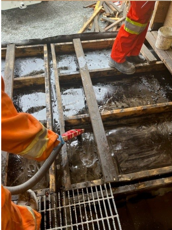
Photo 1 and 2 – Oil containment inside building cleaned
