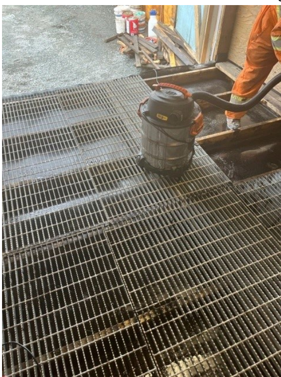
Photo 3 and 4 – Grating and spill tray installed
