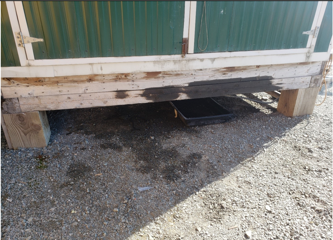
Description: Leaking Motor oil storage for generator.
