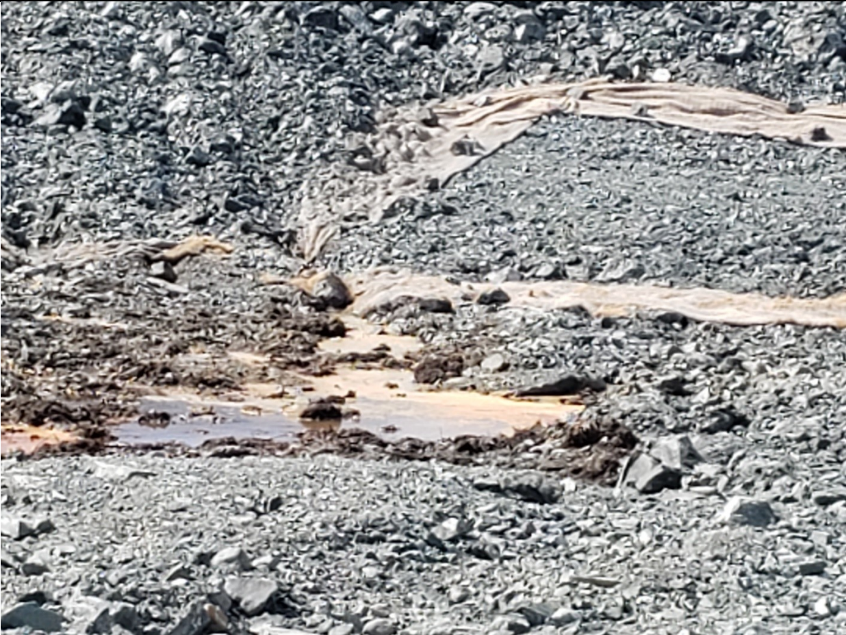
Description: pooling water in the area where the chemical leaching aggregate was used.
