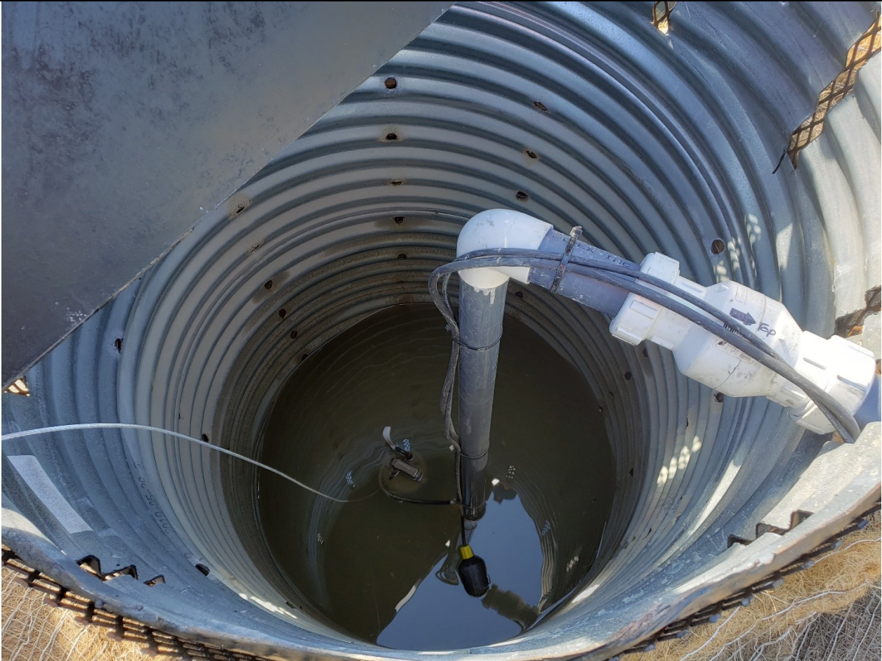
Description: well to designed to capture the leak from the Waste Rock Stockpile
