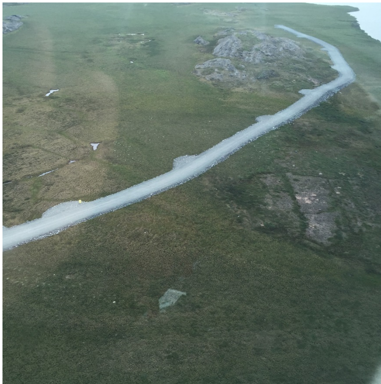
Photo: TIA access road looking southeast – Sampling location 16-QR-04
