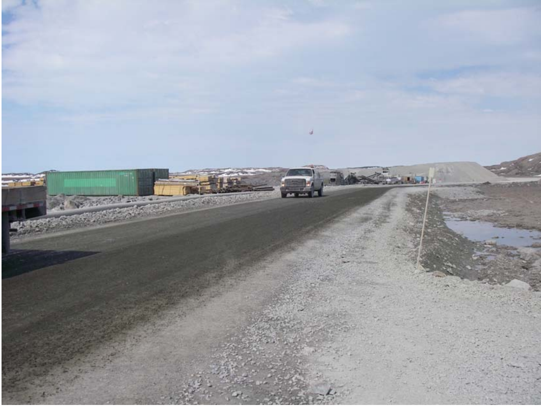
Figure 3 - Road after application of EK-35.
