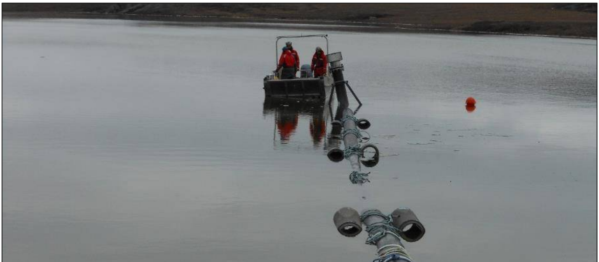
Photo 9: Crew deploying one of the 14" suction for the TIA pumps in the 710 Area.
