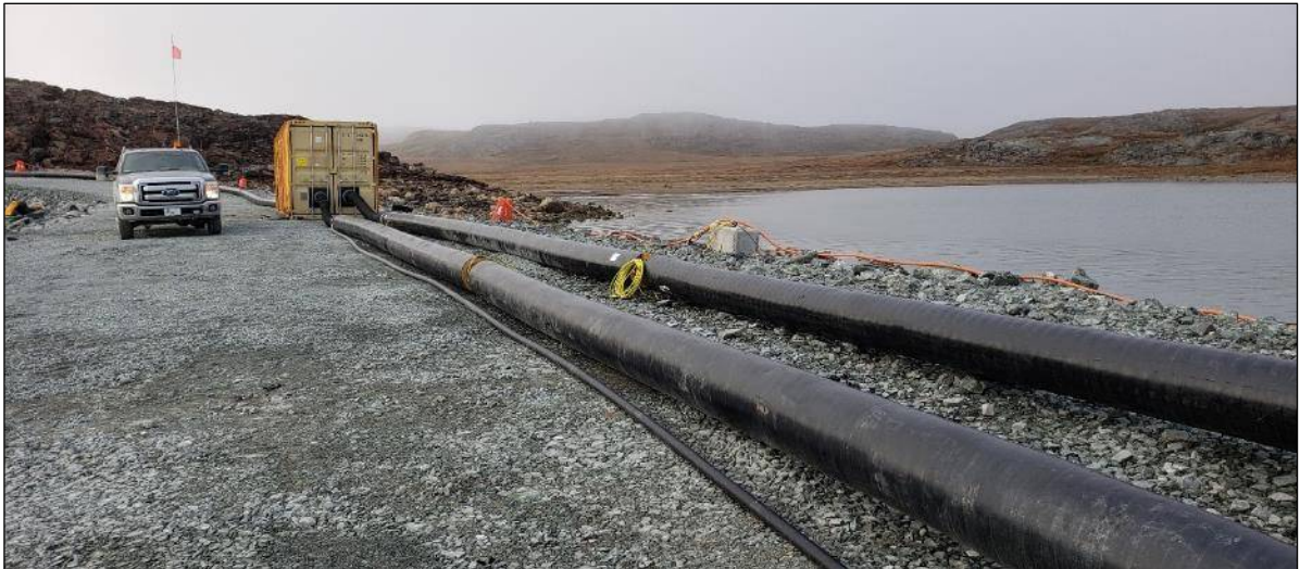
Picture 15: 730 mechanical pump house after connection with intake and discharge pipeline.
