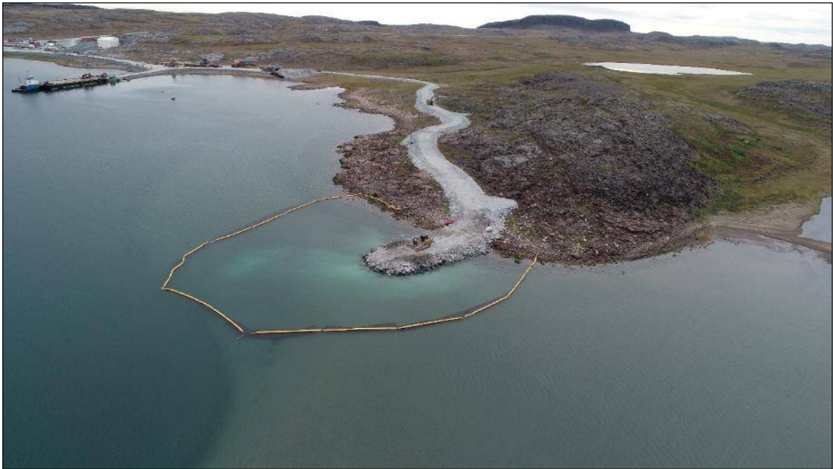
Picture 13: Construction of Marine Outfall Berm and access road. Silt curtains were installed to contain sediments.
