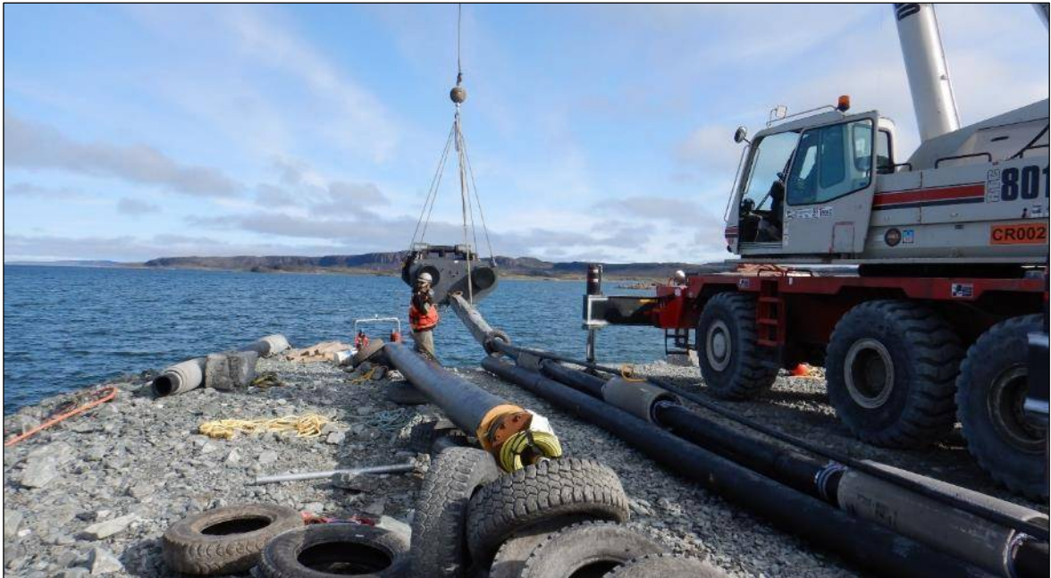
Photo 19: With the help of a crane, deploying the 8" assembly of the recirculation line at the Marine Outfall Berm. Concrete weights are used to submerge the pipeline.
