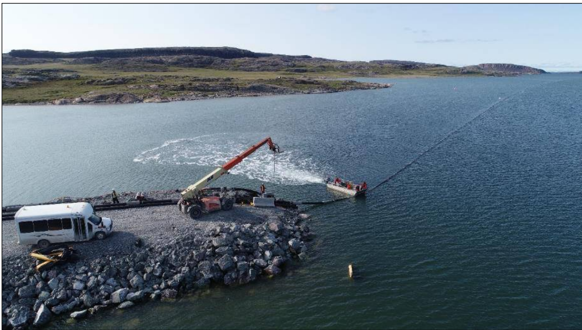
Picture 18: Crew working from Marine Outfall Berm, and a smaller boat for the deployment of the underwater pipeline and diffuser.
