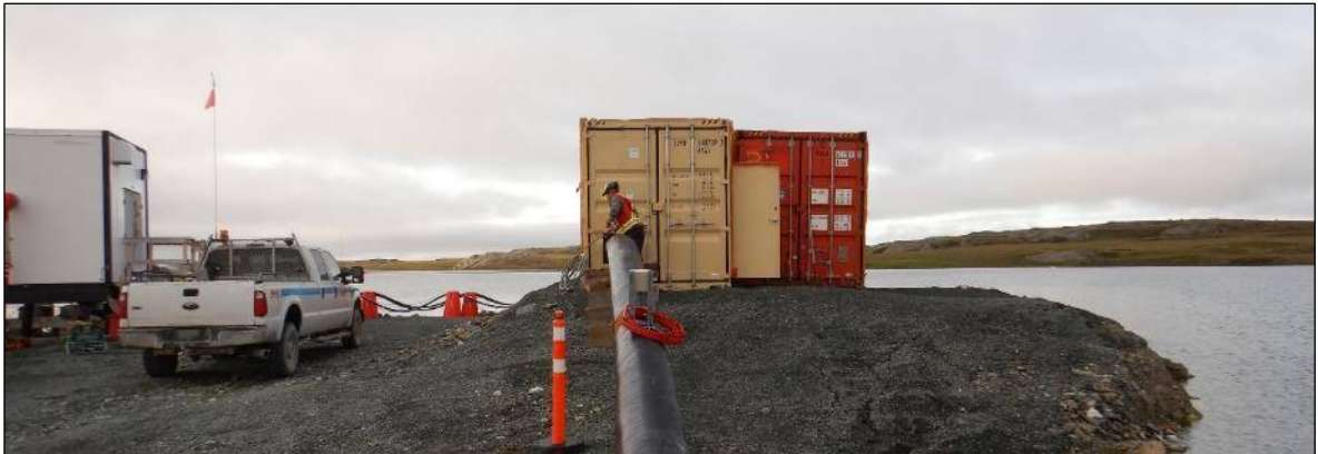
Photo 7: Electrician finalising the installation of heat trace on the 710 pump station. Pumping station in beige, electrical room in red.
