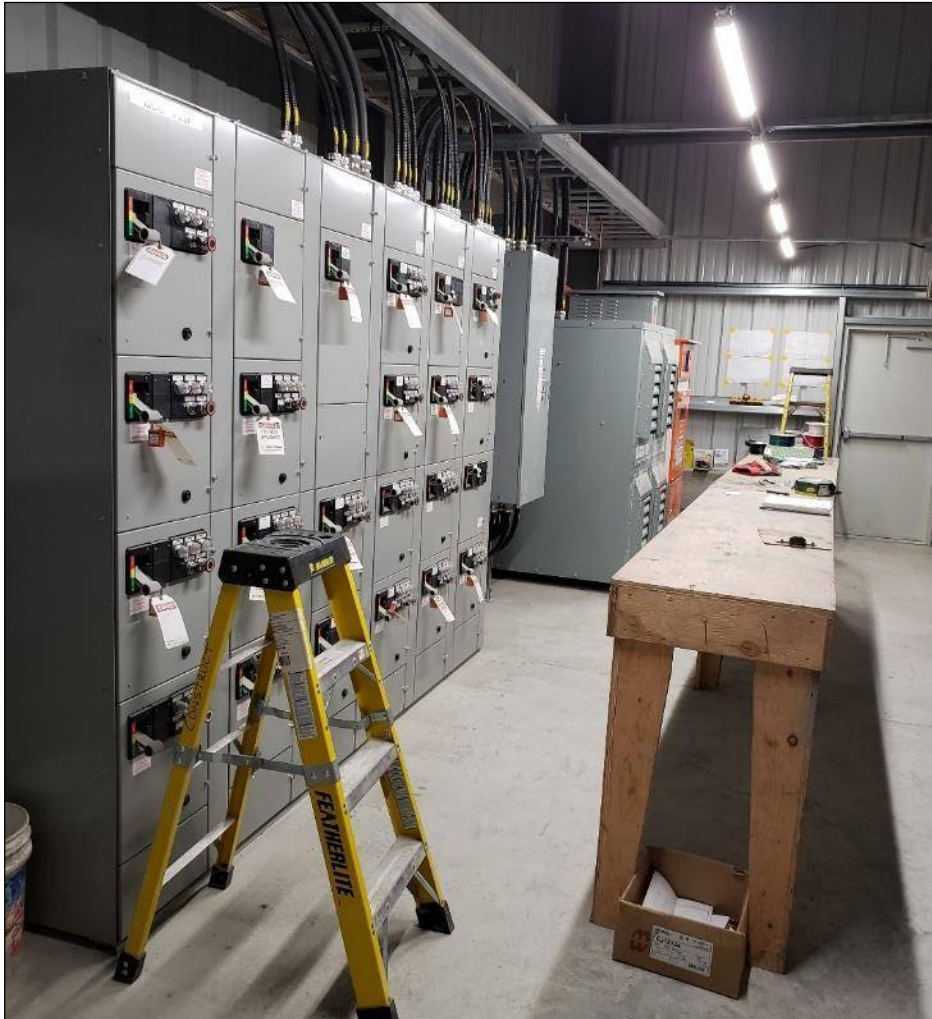
Picture 12: Electrical room in the outfall pumping building (720) during construction, with equipment locked out.
