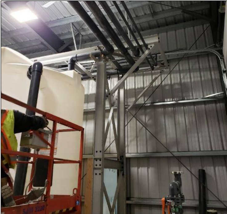
Photo 23: Installation of PVC piping using a scissor lift to connect the Area 740 plant to the 720 building. Outfall discharge pump box showing on the left side (opaque white tank).
