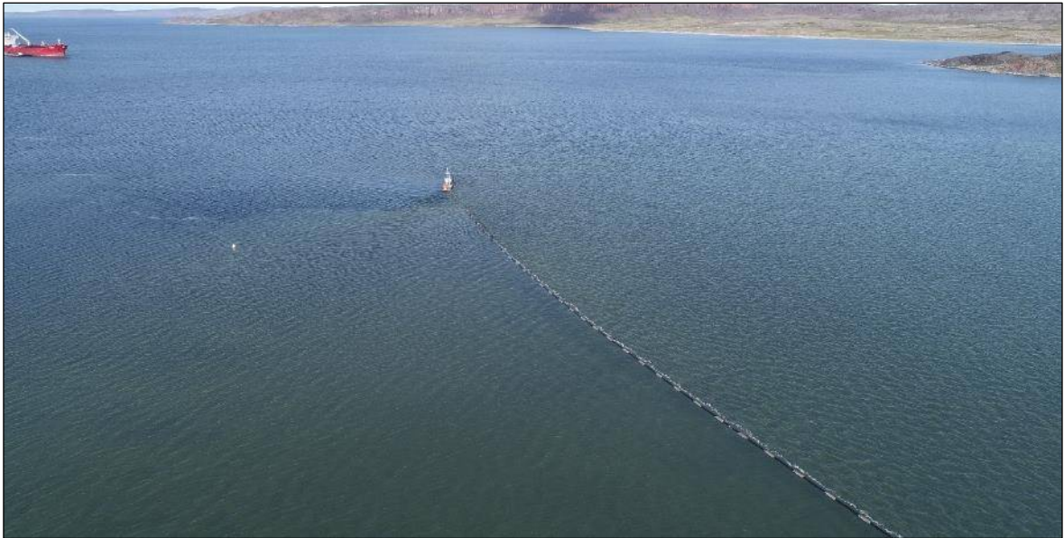
Picture 17: Tugboat keeping tension and controlling the discharge pipeline and diffuser floating on the water surface during deployment.
