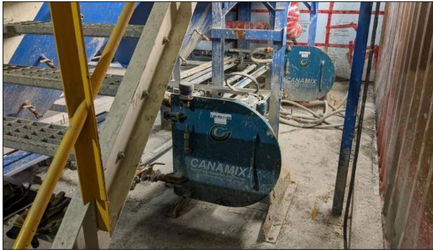
Picture 30: New hose pump installed on new concrete floor in the 740 building, at the underflow of clarifier.
