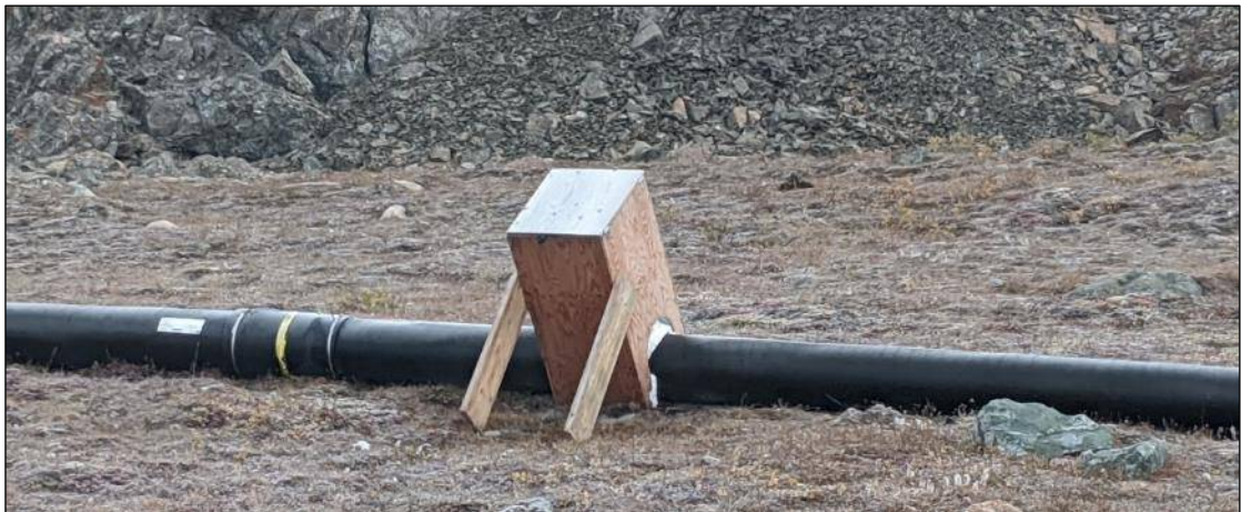
Photo 29: A vacuum breaker with insulated and heated shelter.
