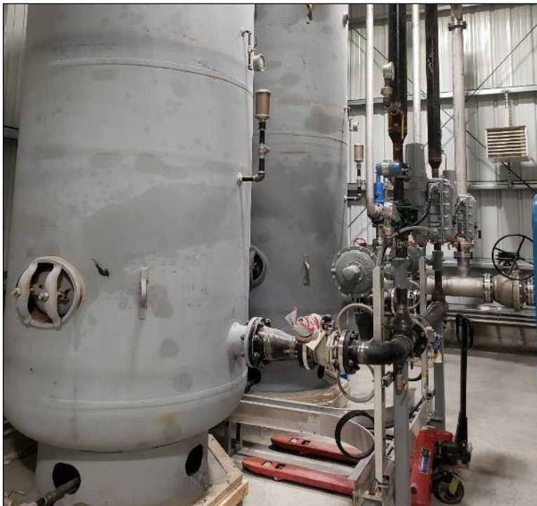
Photo 11: Compressor system for pigging the line installed and ready for commissioning.
