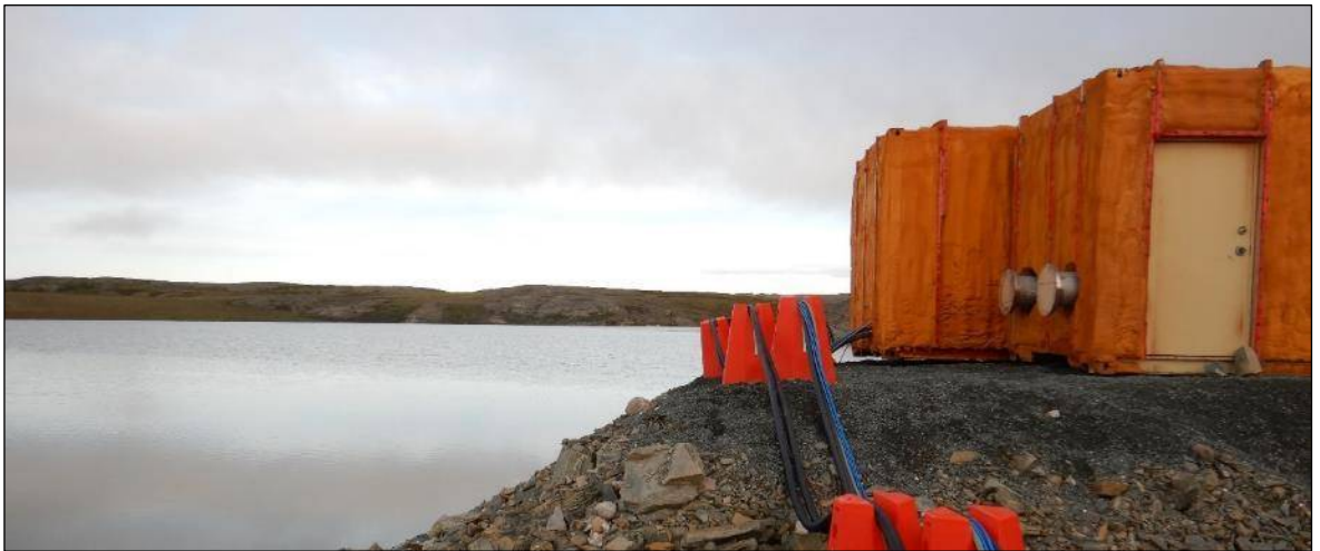
Photo 8: Showing the 710 buildings after insulation. Main power cables coming into the electrical room and the two stainless steel connections for reclaim pipelines.
