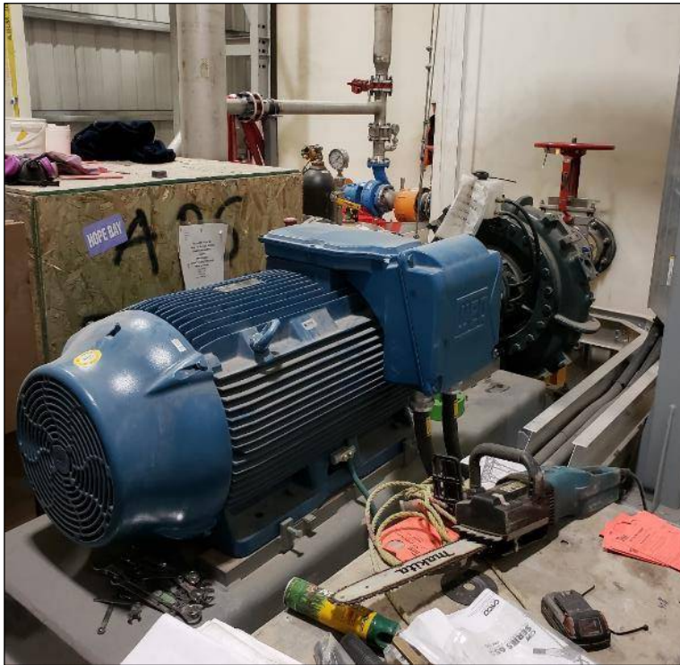
Photo 10: Large outfall transfer pump 720-PU-001 during construction.
