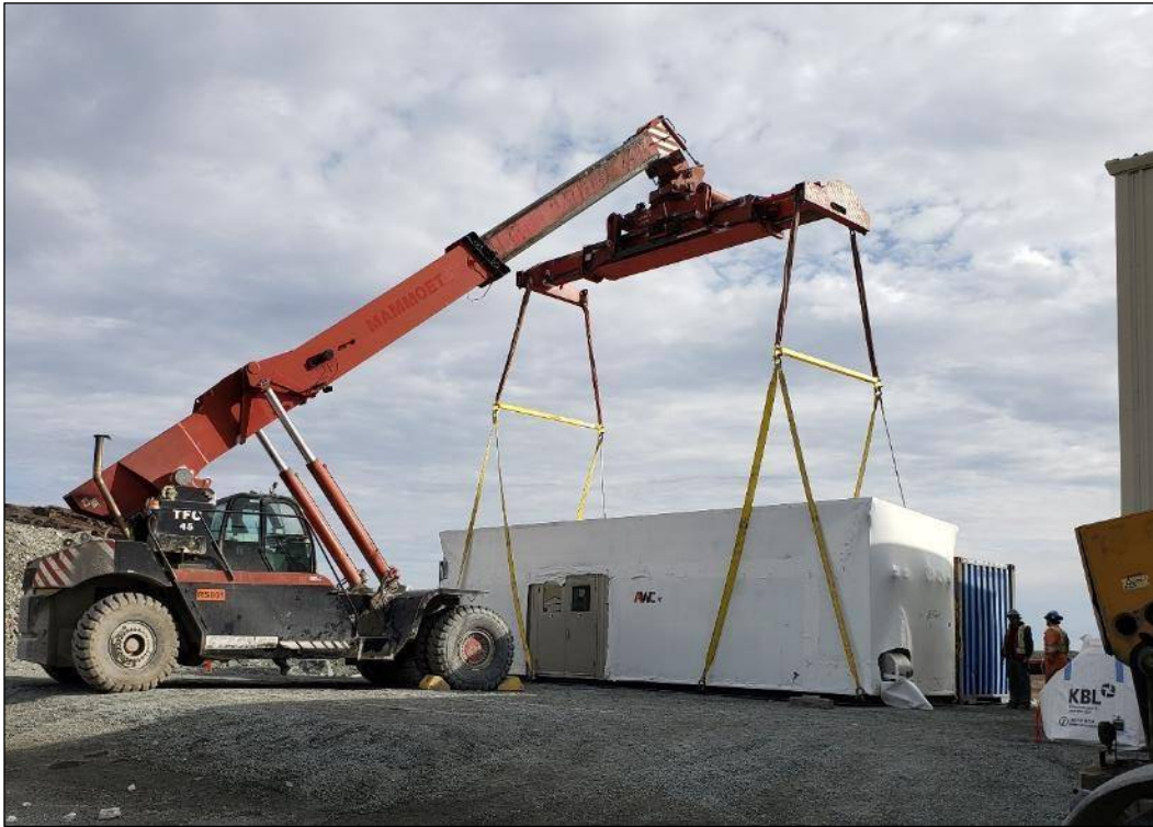
Photo 21: Installation of Area 740 plant supplied by BQE Water, on its pad.
