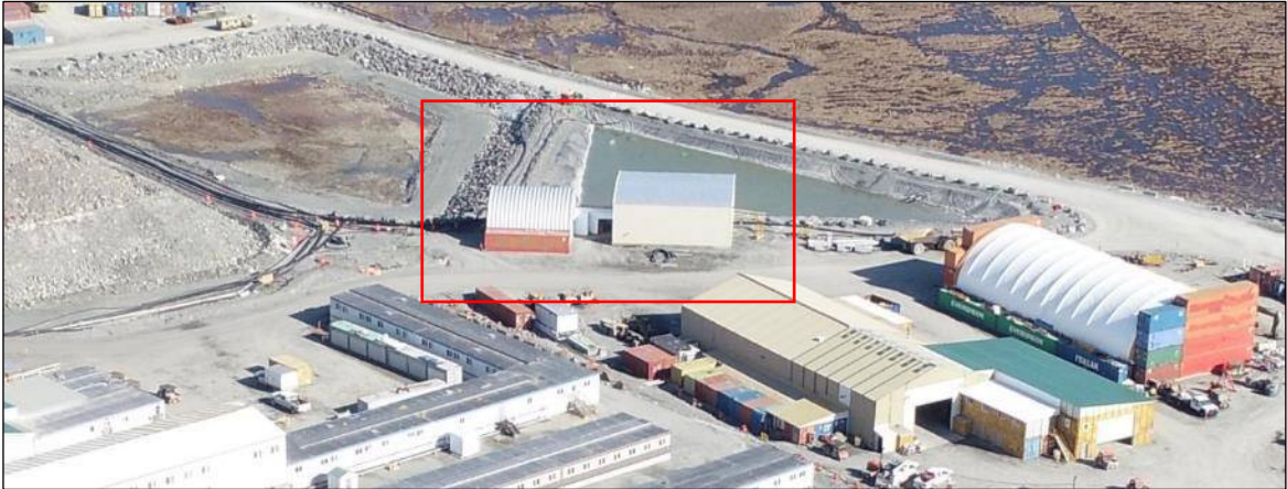
Photo 2: Outfall pumping system (720) and TSS filtration plant (740) next to the sediment pond. 720 in beige on the right and 740 in orange/white on the left.
