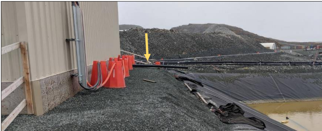
Photo 27: Showing the new overflow pipe coming from the concrete foundation of the 720 building into the sedimentation pond.
