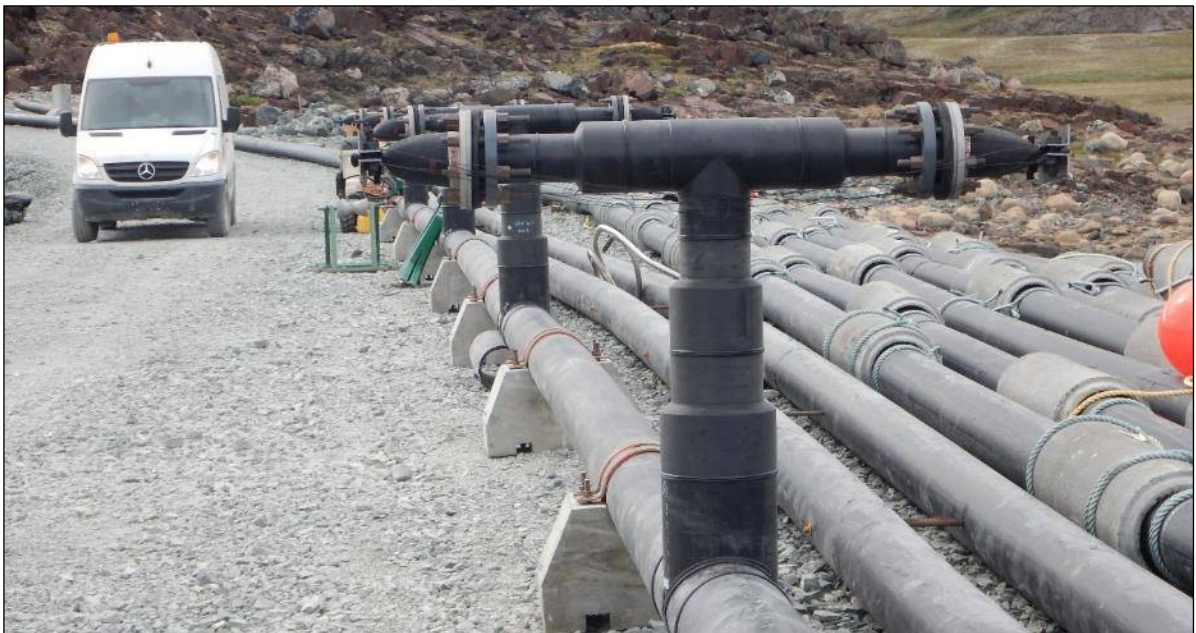
Picture 16: Showing fully assembled diffuser and 200' sections of weighted pipe ready to be deployed and staged on the Marine Outfall Berm and access road.
