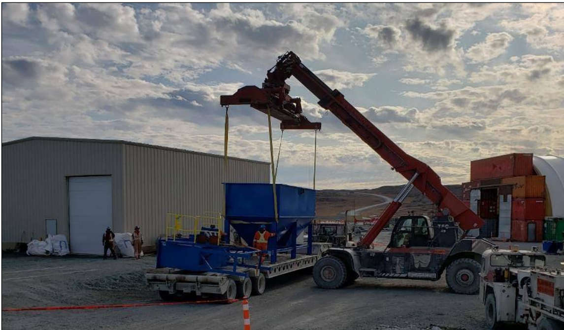
Photo 22: Offloading Area 740 clarifier from truck prior to installation.
