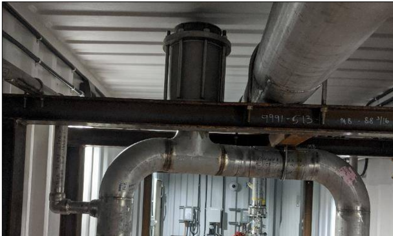
Photo 25: Showing new air release valve installed in the 710 Building.
