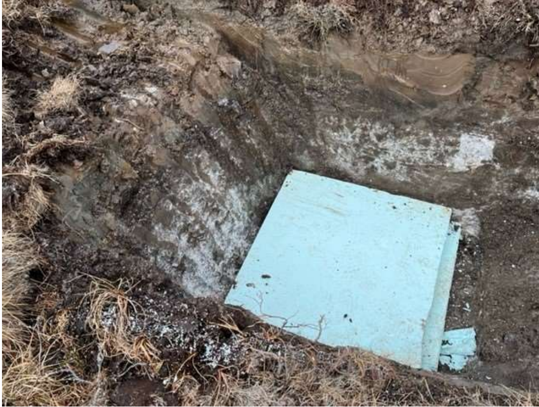
Photo 2 - Excavation completed, and rigid installation installed to the base of the excavation. Excavation side slopes were carefully cut to the required dimensions with an excavator equipped with a ditching bucket.
