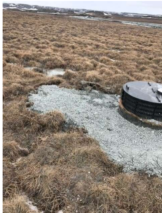
Photo 4 - Backfill with bedding material is complete.
