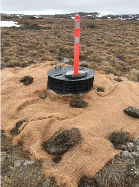
Photo 5 - Sump installation complete. Lid placed on top of sump to remove hazard to humans and wildlife. Coconut matting placed over bedding material.
