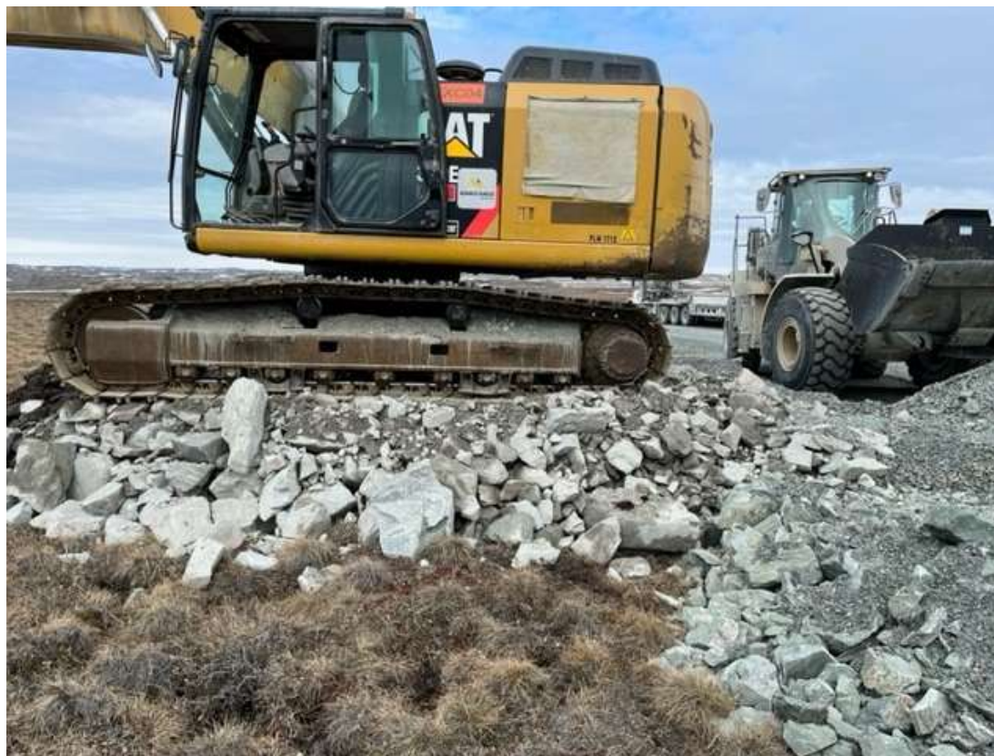
Photo 1 - Pad constructed with non-acid generating ROQ for equipment access from Windy Road to the sump location
