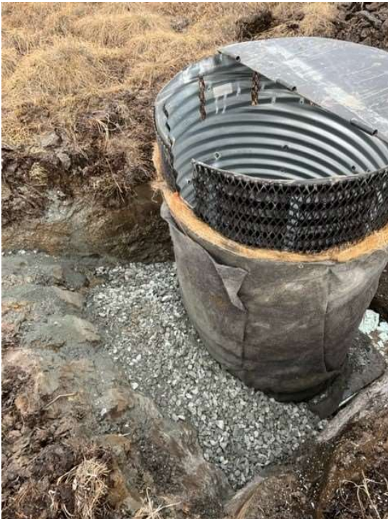
Photo 3 - Sump and non-woven geotextile installed. Backfill with bedding material in progress. The liner bedding material was placed in lifts.
