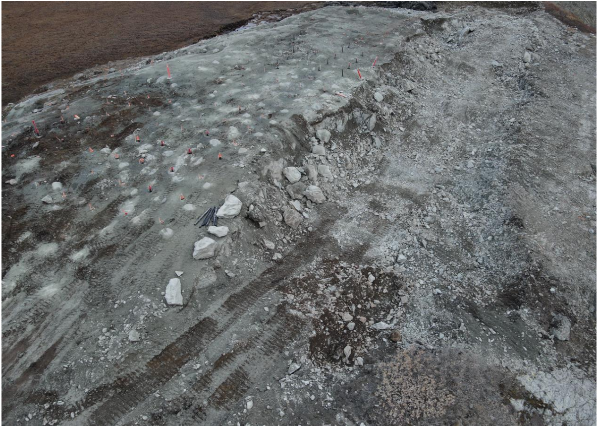
Pad Construction – Drill and Blast
