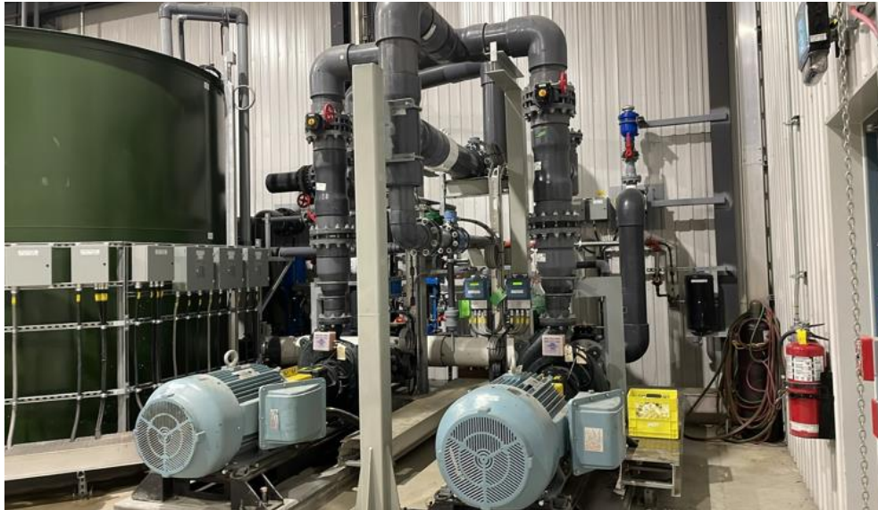
Treated Water Tank and Pumps
