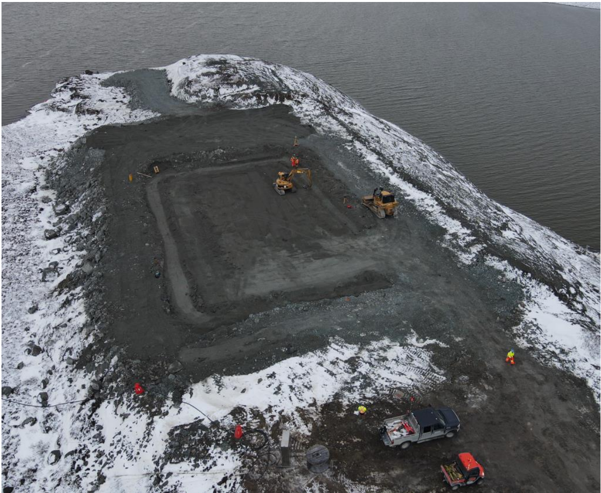
Pad Before Final Levelling – Building footing excavation
