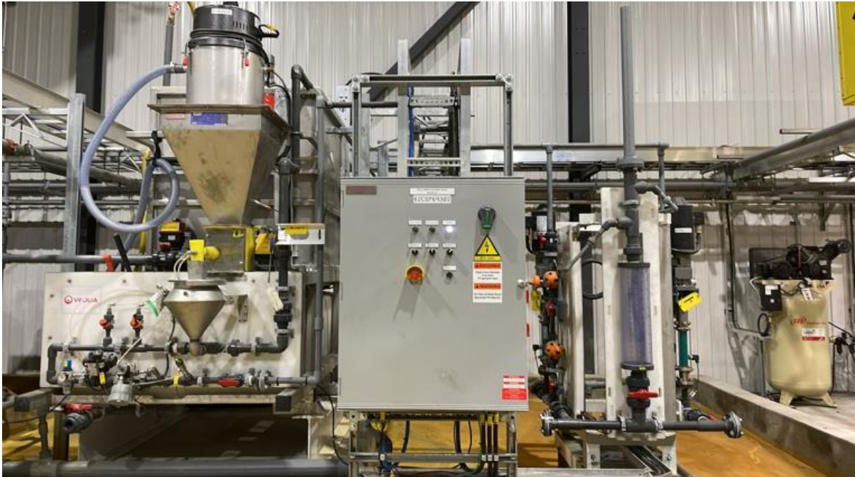
Polymer Makedown and dosing Skid
