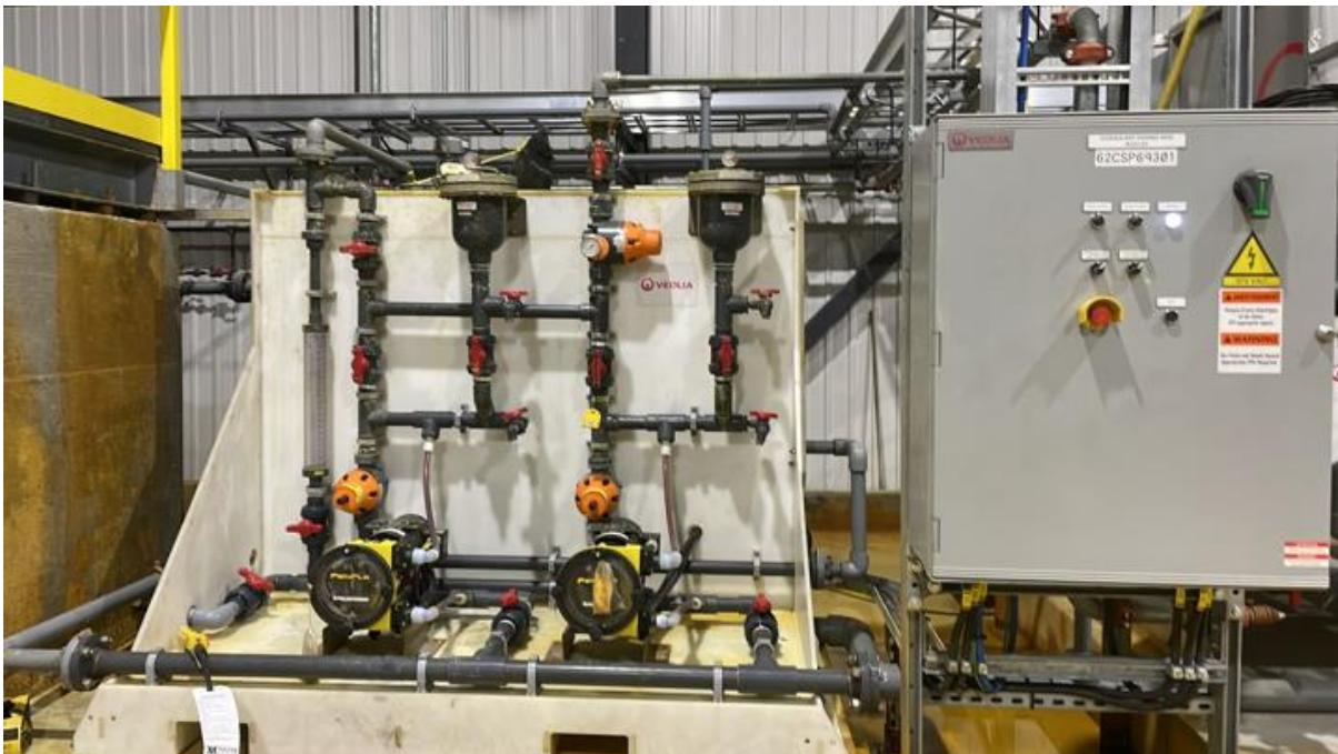
Coagulant Dosing Skid
