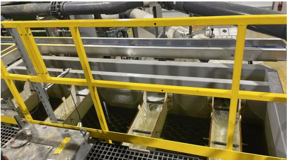
Treated Water (Actiflo Overflow)
