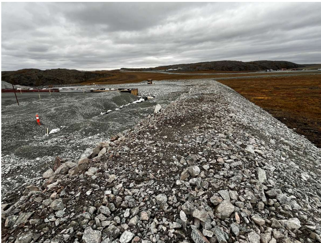
Photo 6 Non-Contact Berm Completed Protection
