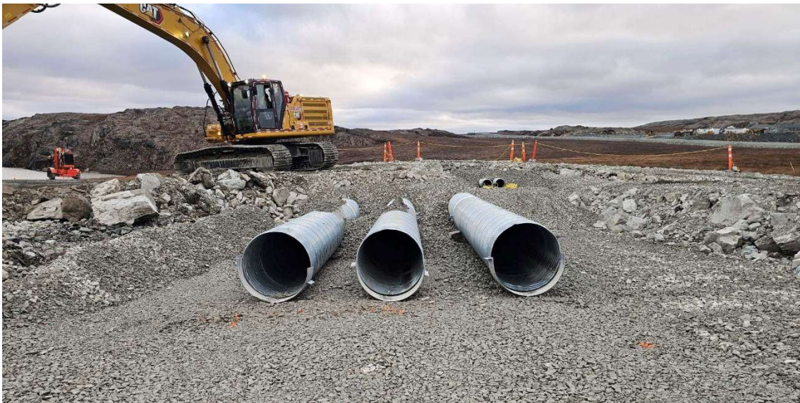
Photo 7 Non-contact Culvert Installation
