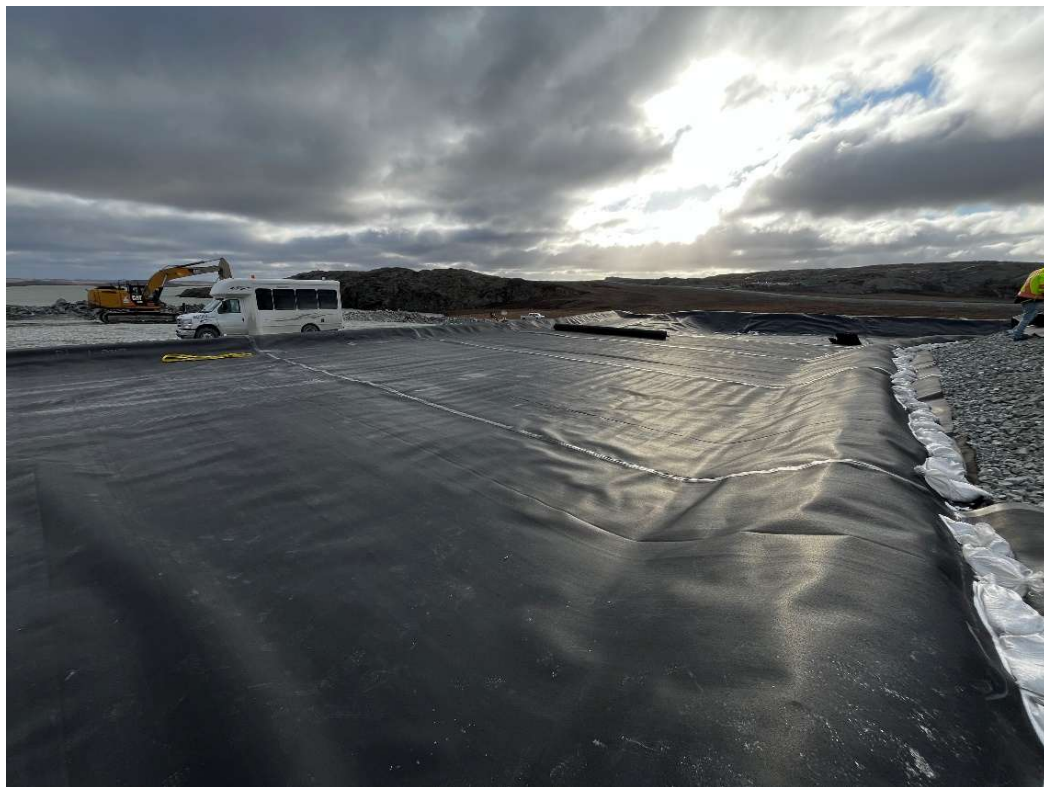
Photo 10 Fuel Storage Secondary Containment Liner Installation
