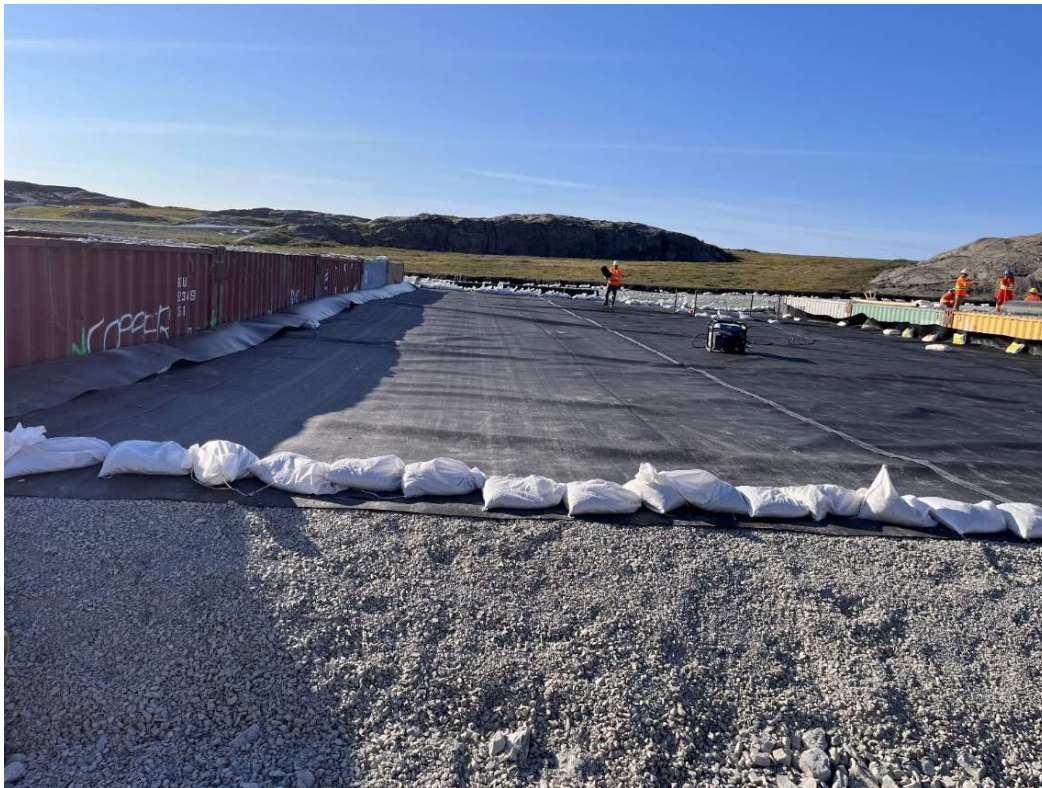
Photo 1 Maintenance Dome HDPE Liner Installation
