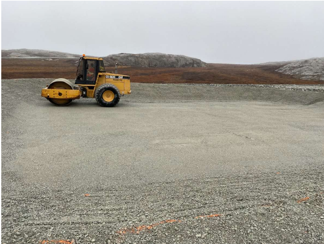
Photo 9 Fuel Storage Secondary Containment Preparation
