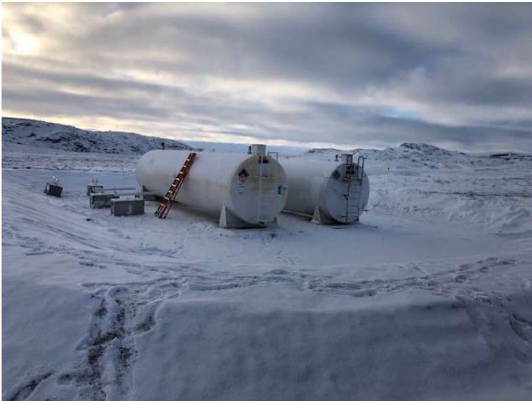
Photo 12 Fuel Storage Secondary Containment Tank Placement
