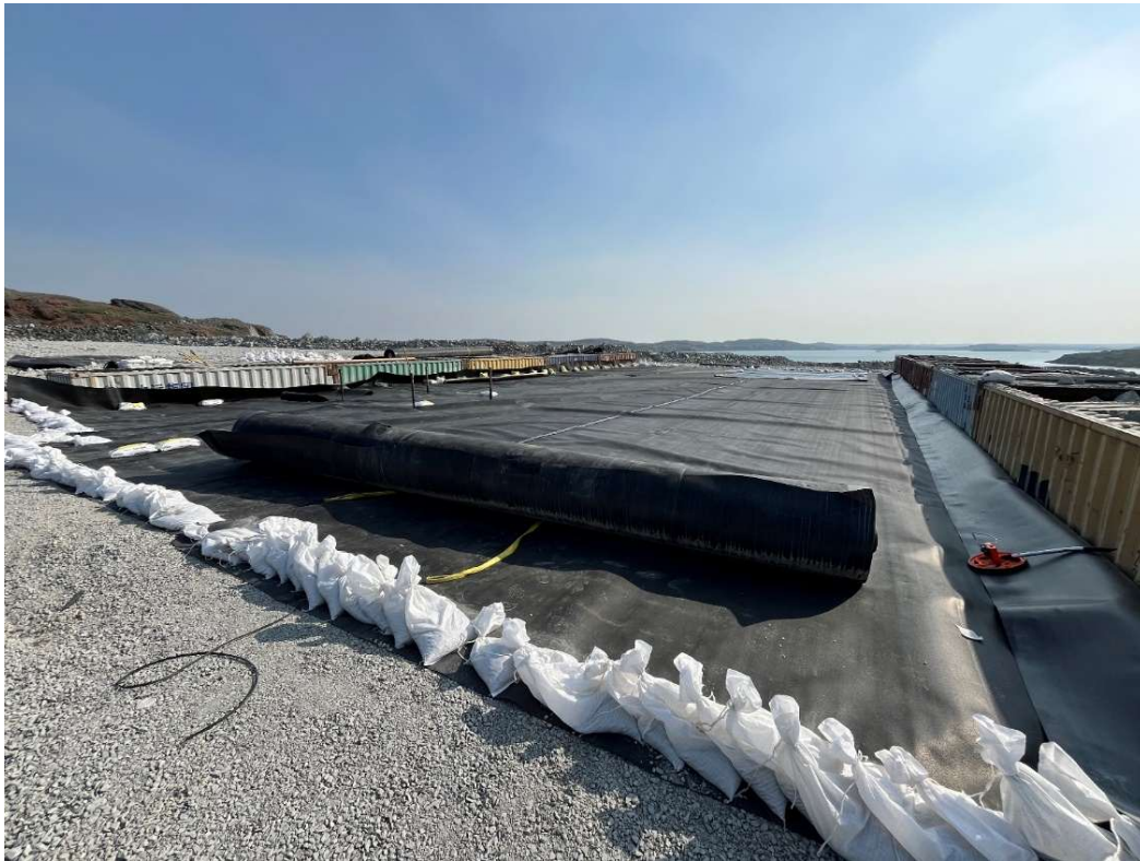
Photo 2 Maintenance Dome Geotextile Liner Protection
