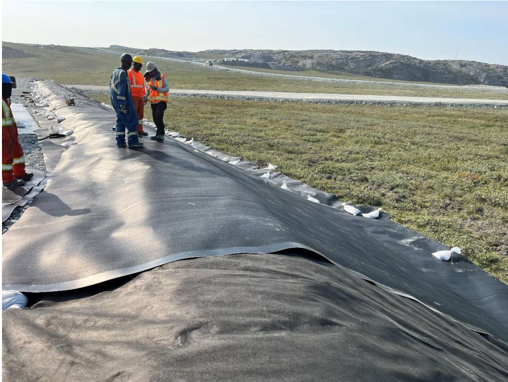
Photo 5 Non-Contact Berm Liner Installation
