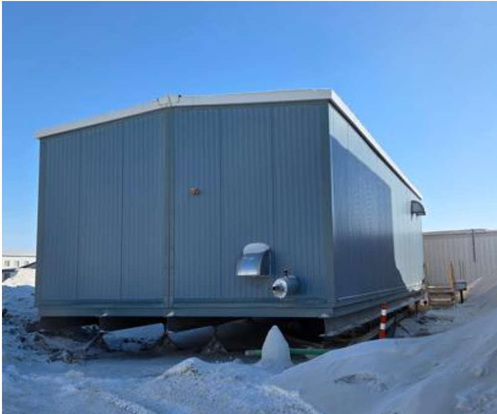
Building installation completed
