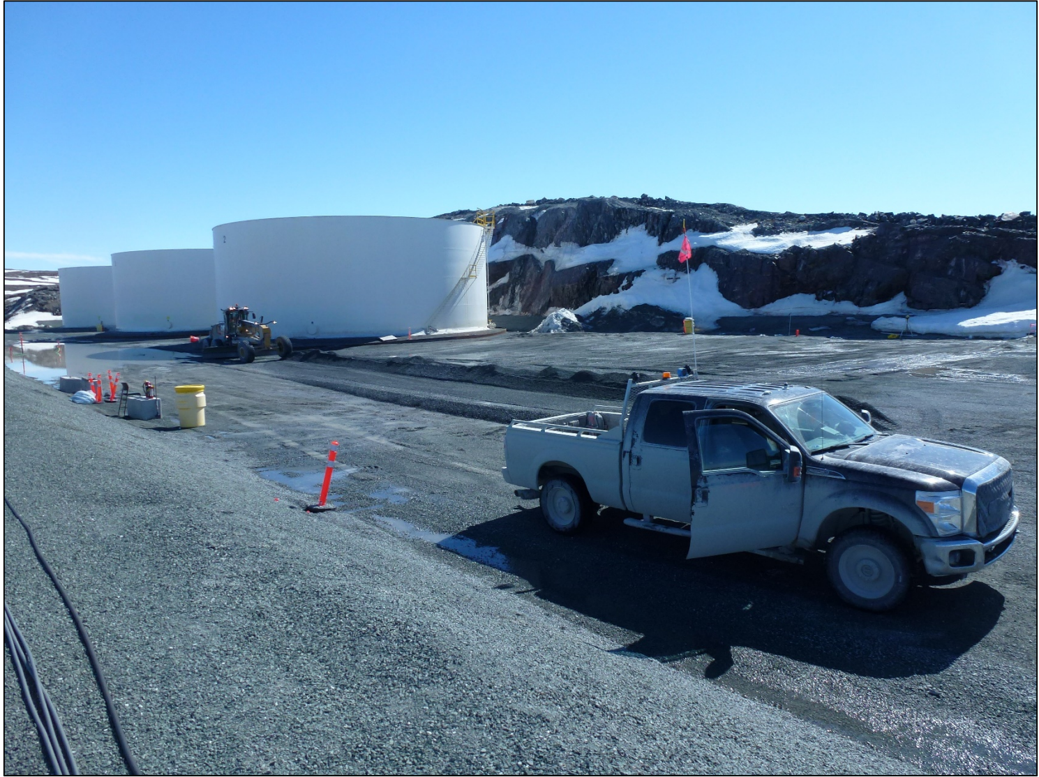
Topping up liner cover with crush material (June 13, 2019)
