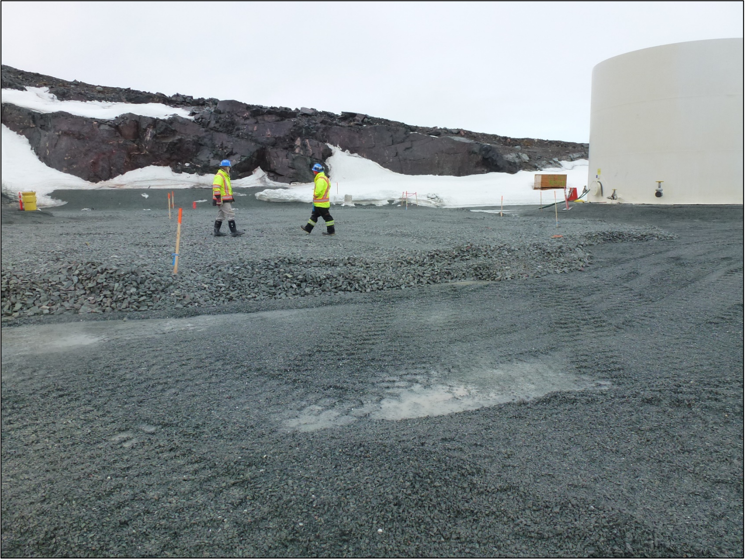
Placing base of 3 inch minus material for tank pedestal (June 14, 2019)
