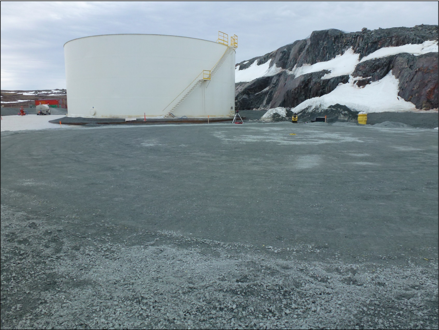
Compacted final surface of pedestal for Tank No. 1 (June 17, 2019)
