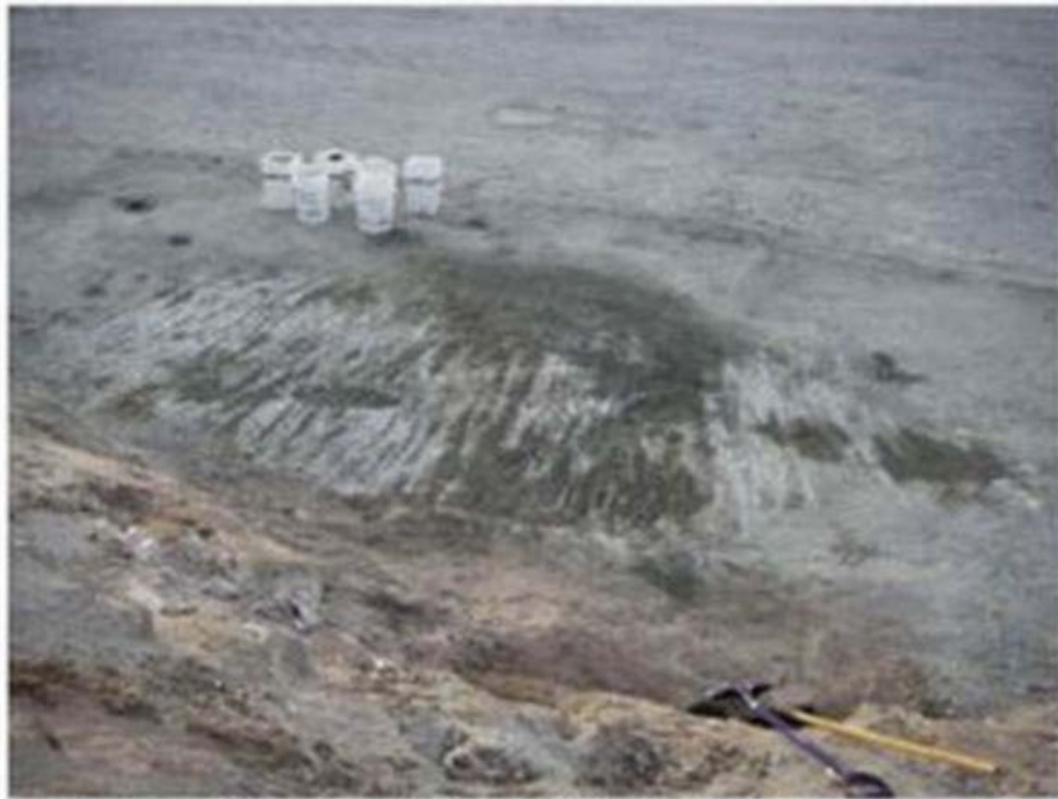
Photo 5: The surface of the frozen material in the area of the glycol spill was scraped up with the teeth of the excavator. The material was placed in buckets to be taken to the Waste management Facility for proper disposal.
