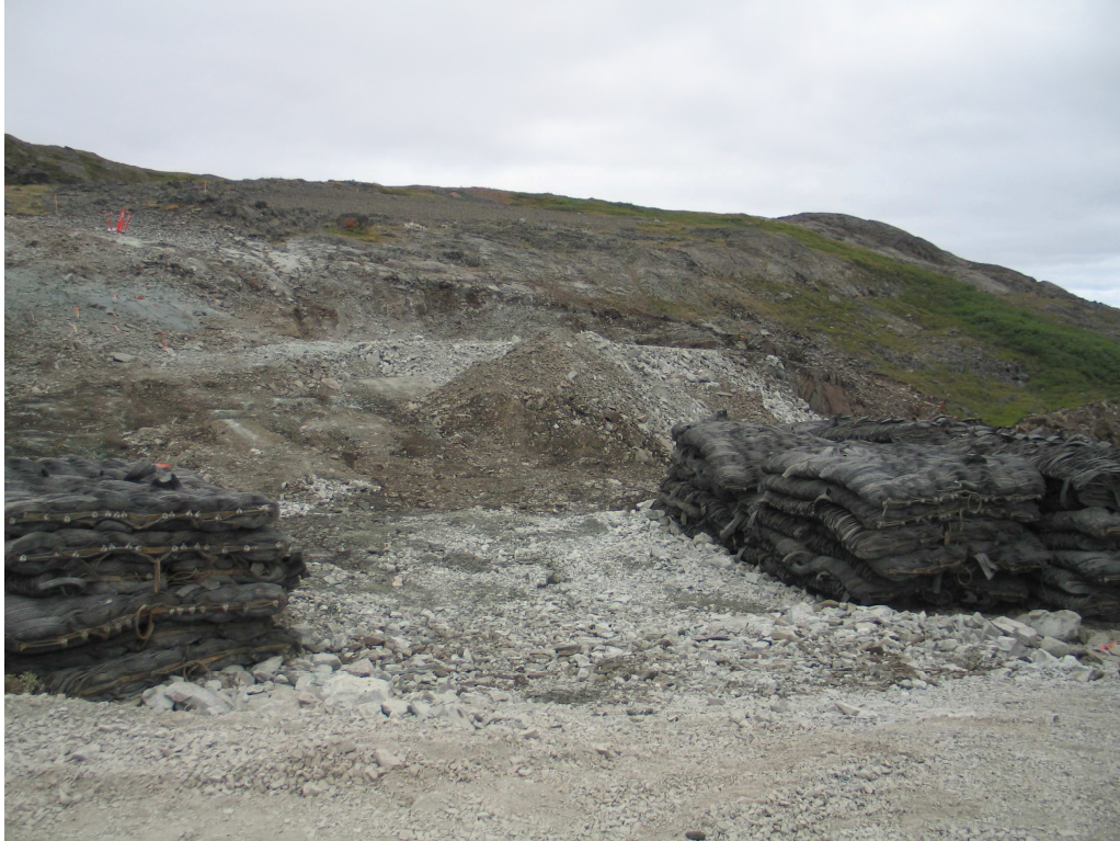
Photo 6: Placing ROQ on the Fuel Transfer Access Road at start of turn around.
