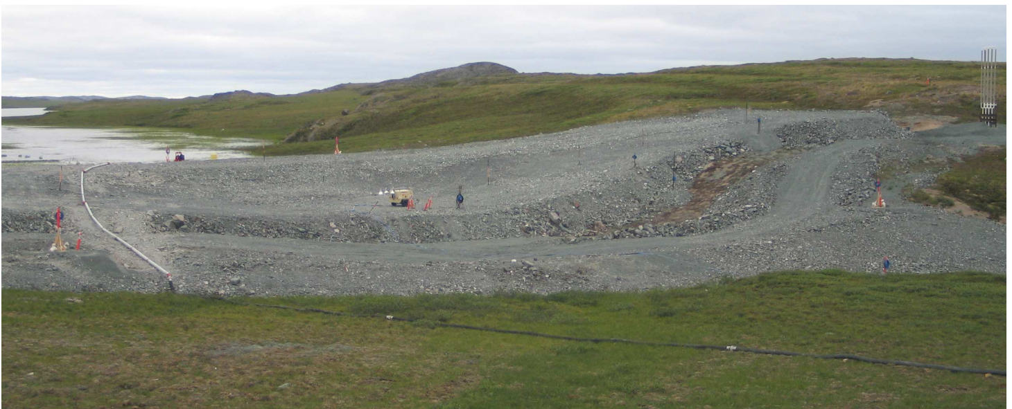
Photo 2: North dam, showing pipeline and some of the raised multi bead cables.
