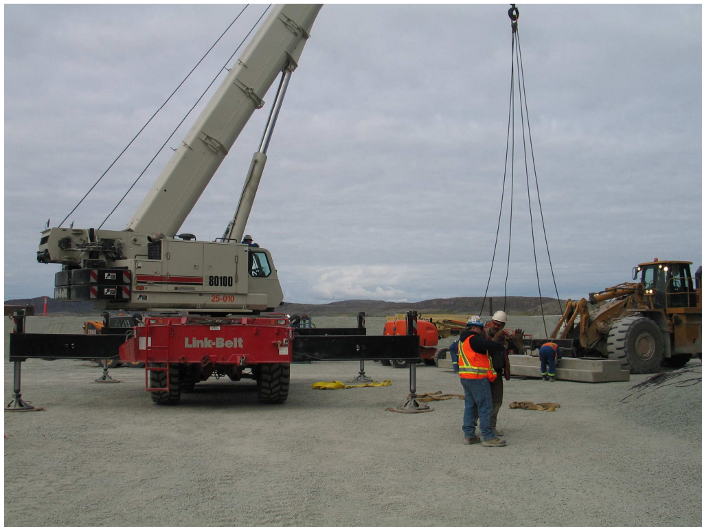
Photo 8: Weighing bridge sill with the crane. Weight is 28,900 lbs.
