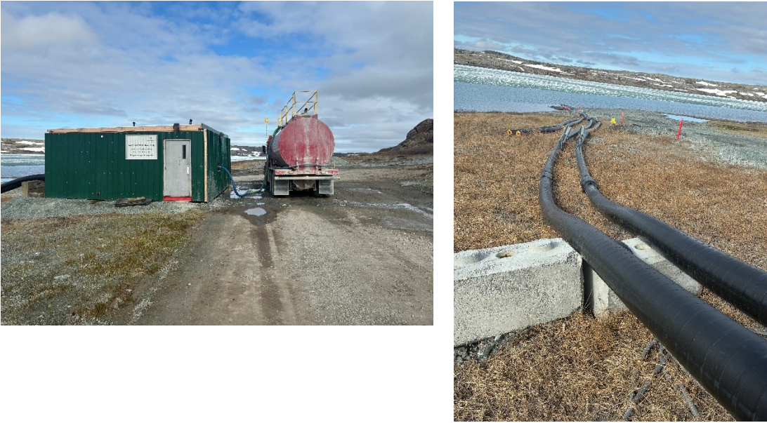
Figure 1-2: Existing Fresh Water Intake Facility
