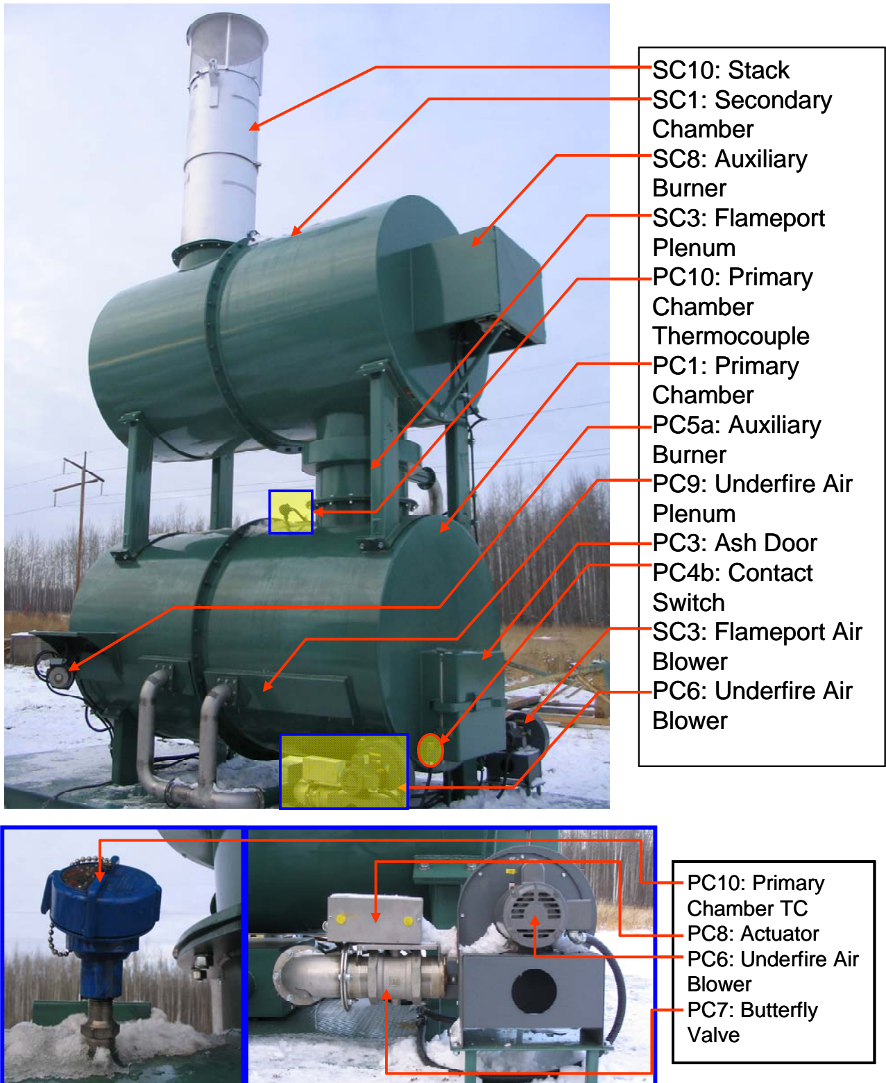
Figure 7 Components in the Primary and Secondary Chamber Sections (2)
