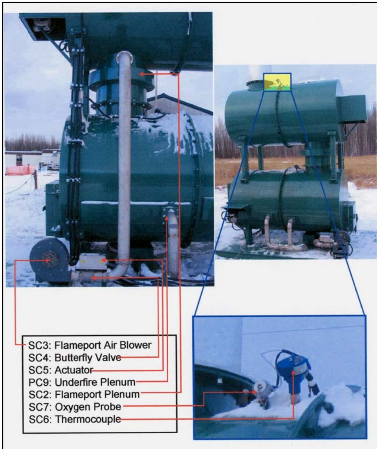
Figure 3: Major Components of Primary & Secondary Chambers - Model CY-100-CA-D-O Incinerator
