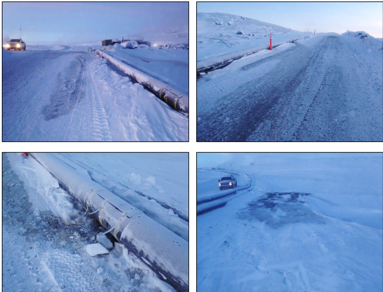
Figure 3. Lake Water Released from Tailings Line During Commissioning
