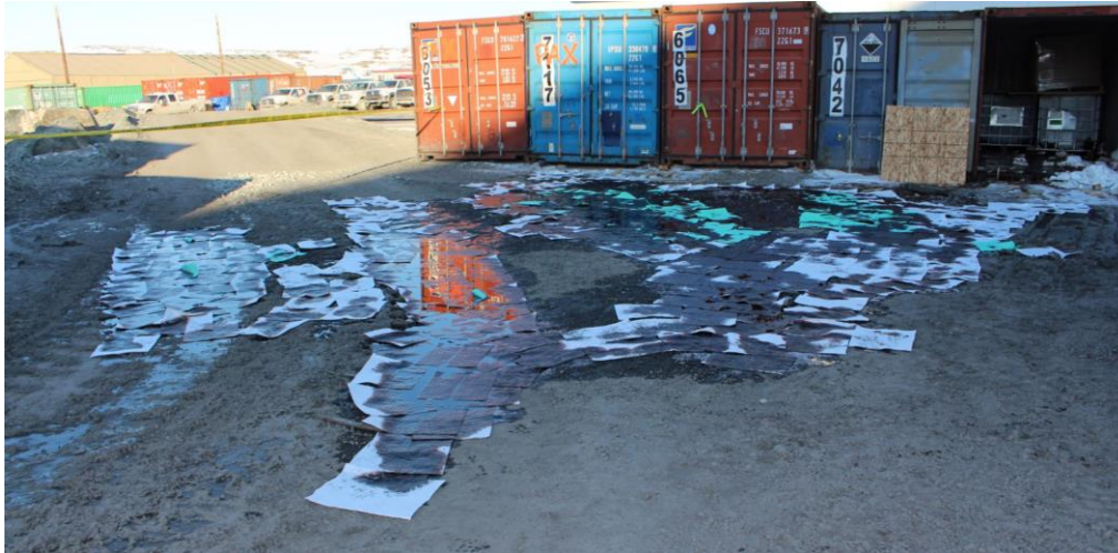
Figure 3. Extent of DanaFloat 245 migration outside storage sea-can and placement of spill absorbent pads.
