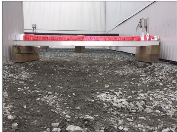
Spill location post-cleanup. Pipeline now fully supported.
