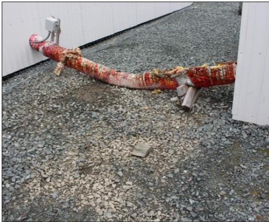
Spill location showing damaged pipeline and cribbing.
