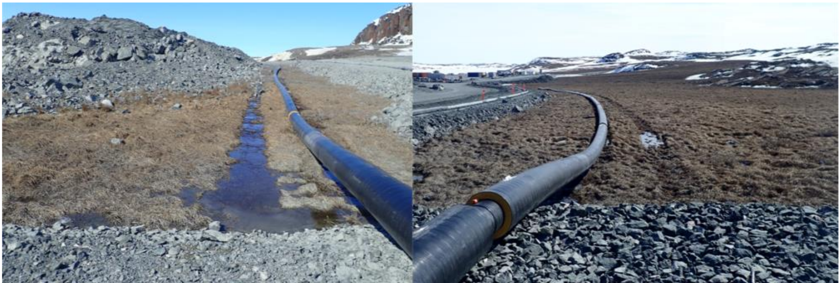
Figure 6. Check dam upstream (left) and downstream (right). Check dam effective in slowing runoff and eliminating turbidity
