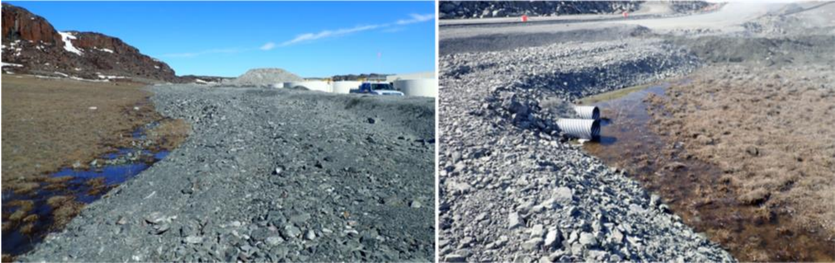
Figure 6. Check dam upstream (left) and downstream (right). Check dam effective in slowing runoff and eliminating turbidity
