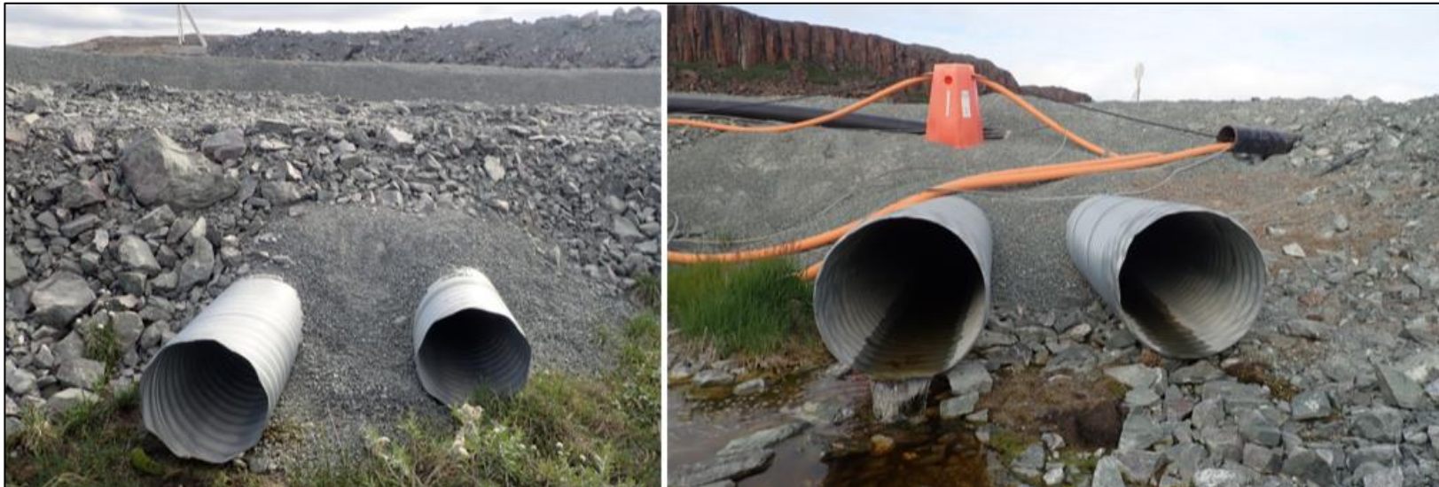
Figure 6. Diversion Berm culverts. Reduced flow observed in July compared to June
