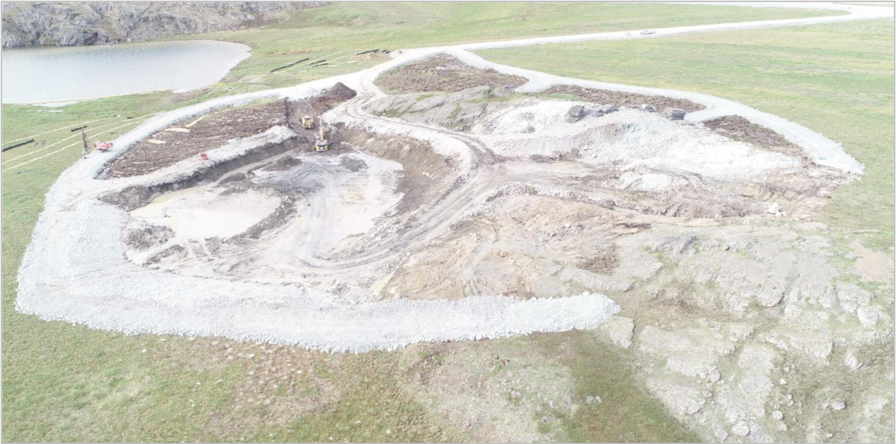
Figure 2. Overburden Stripping at Naartok East Crown Pillar Recovery Trench, July 2019
