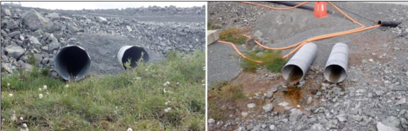
Figure 6. Diversion Berm culverts. Reduced flow observed in August
