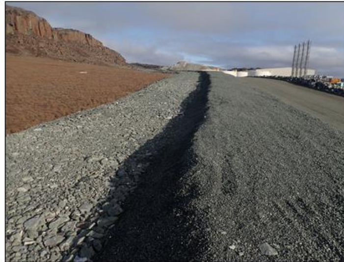
Figure 5. Diversion berm dry during September (left) towards culverts (right)
