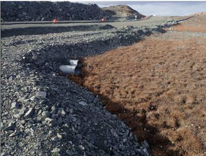
Figure 6. Diversion Berm culverts. Reduced flow observed in September
