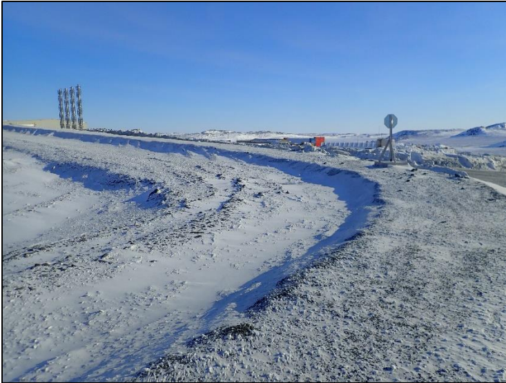
Figure 3. Diversion berm during March 2021
