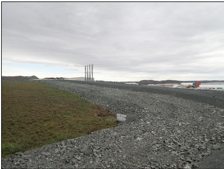
Figure 3. Diversion berm during July 2021
