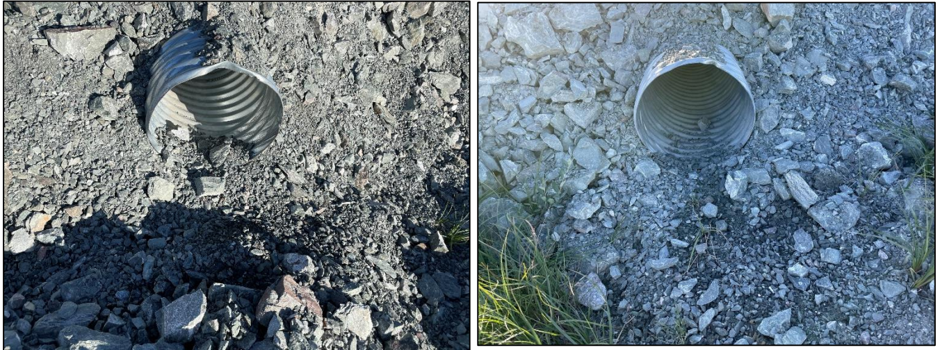
Figure 5. Culvert at km 8 on Madrid All-Weather Road at Naartok intersection upstream (left) and downstream (right) August 2022
