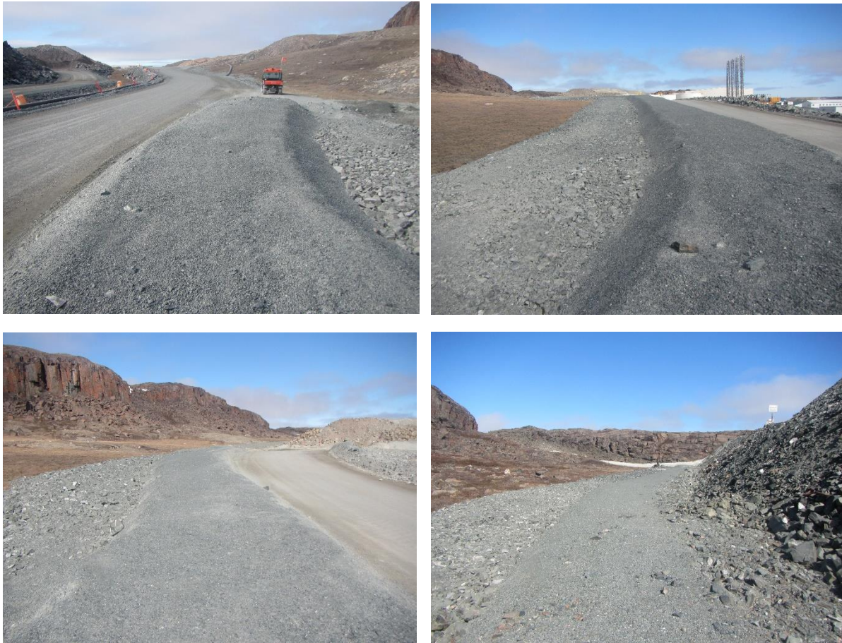
Figure 3. Diversion berm during June 2023
