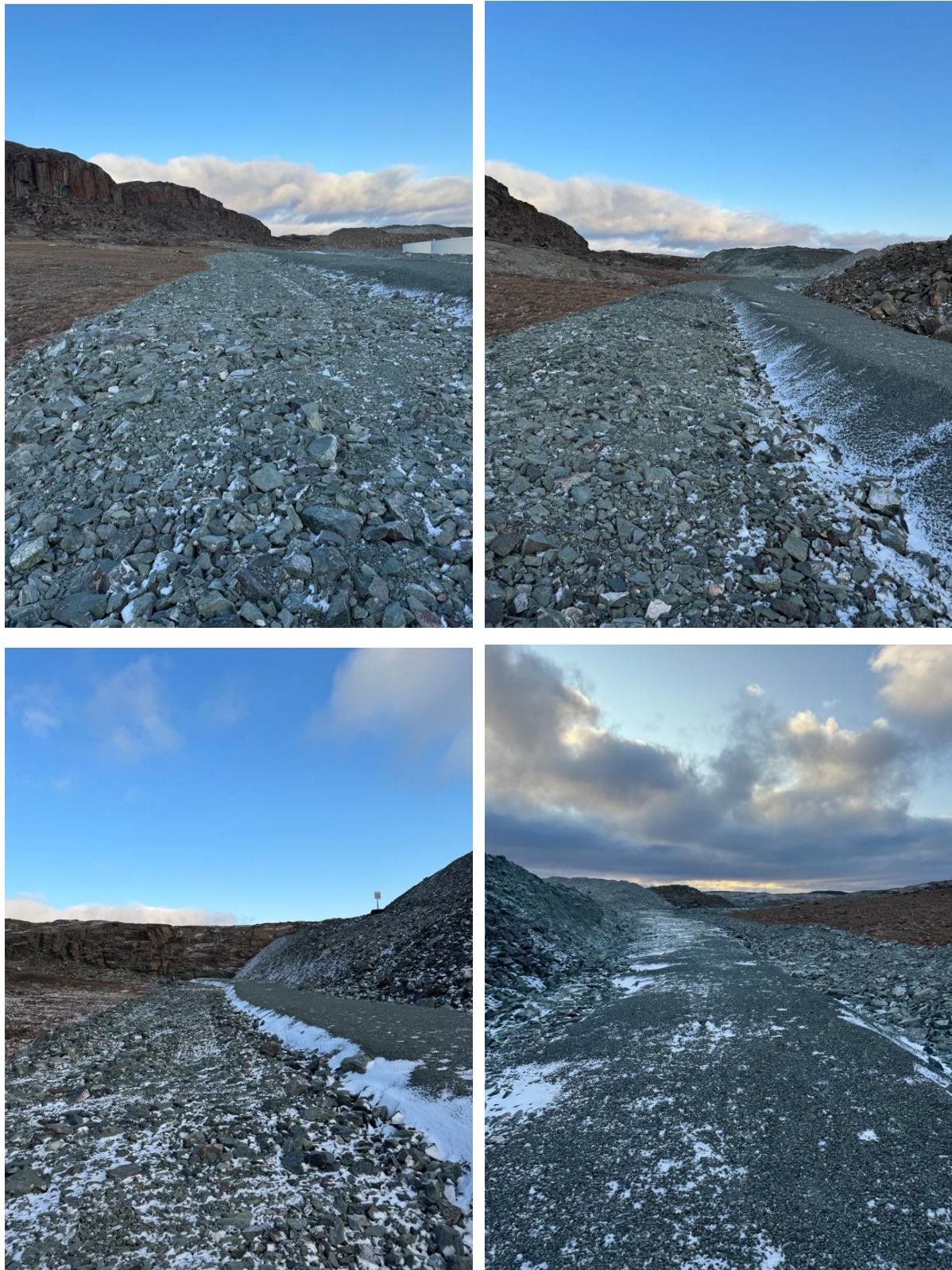
Figure 3. Diversion berm during October 2023
