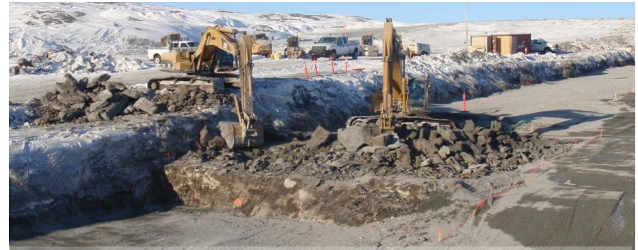
Hyper-saline overburden excavation 'soft spot'
