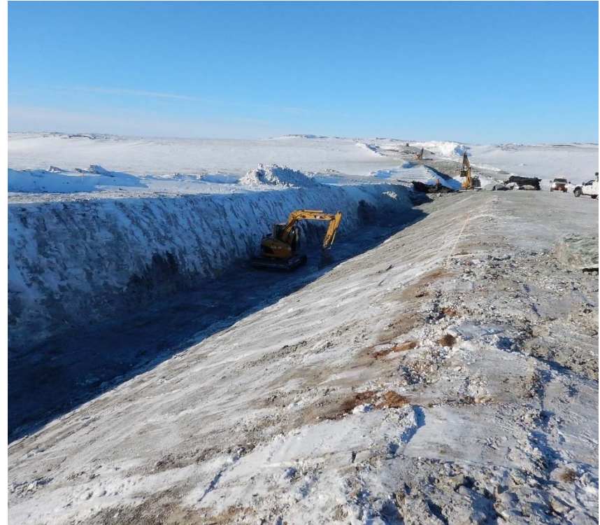
Near complete section of key trench
