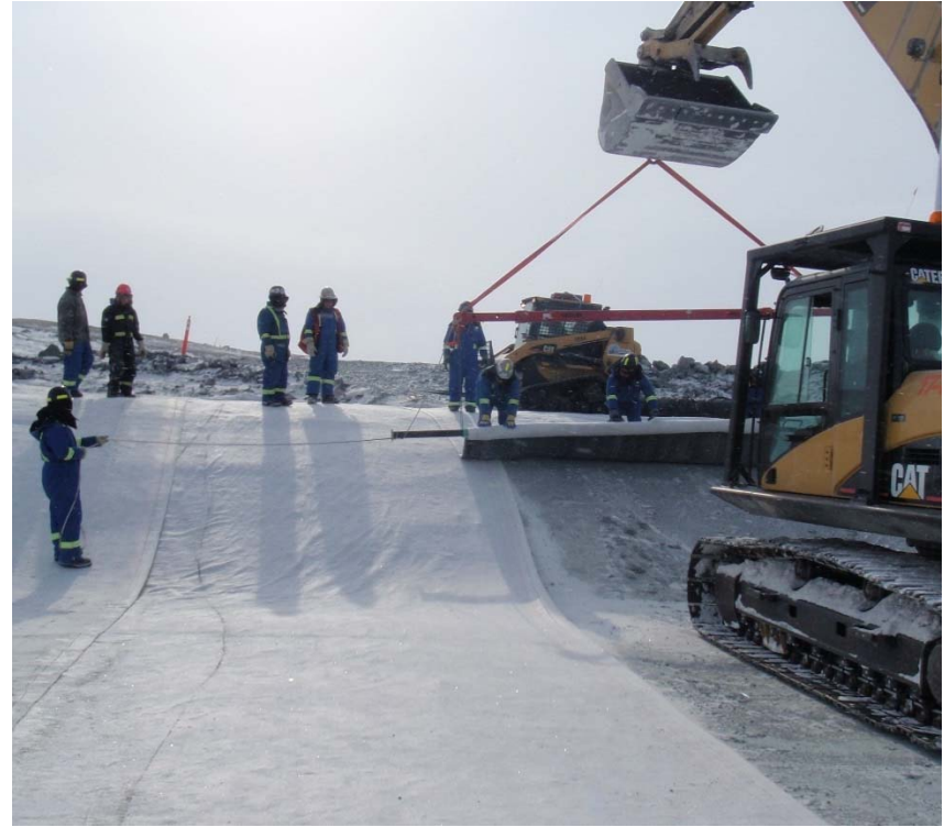
Liner installation in key trench
