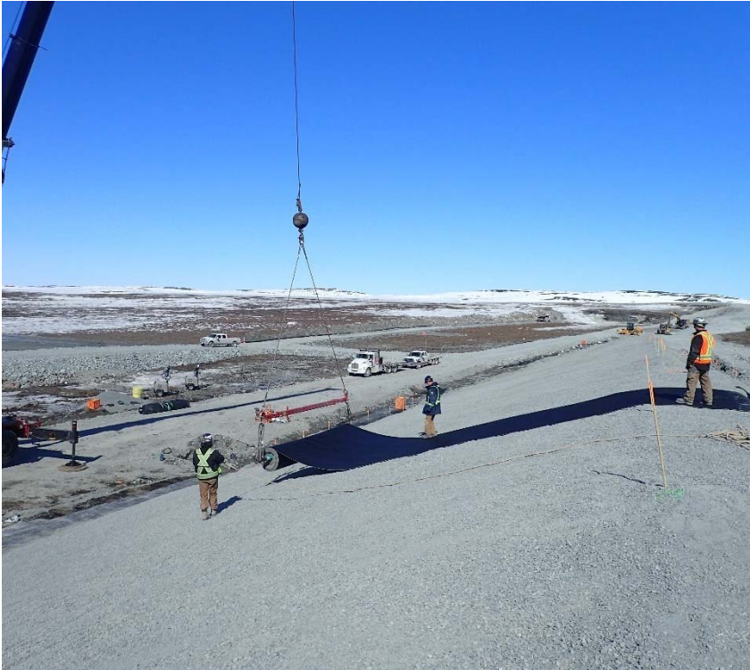
Deployment of liner on upstream slope of above ground fill
