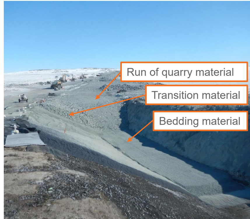
Backfilling of key trench above liner
