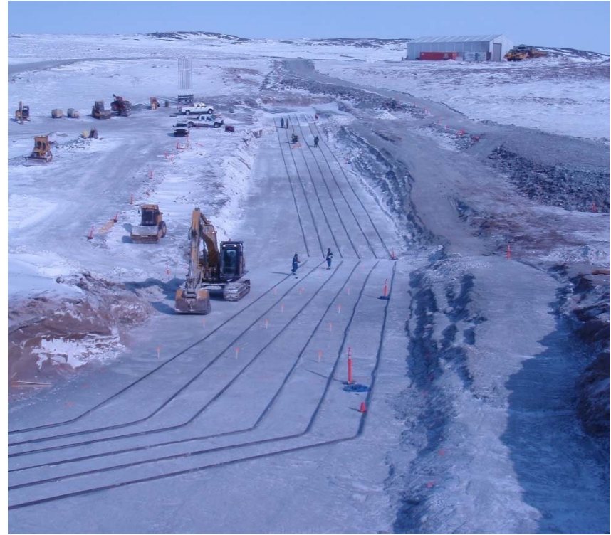
Thermosyphon evaporator pipes installed along the key trench base
