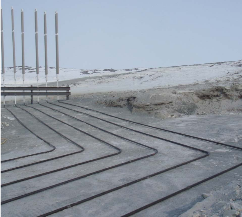
Thermosyphon evaporator pipes connected to radiator
